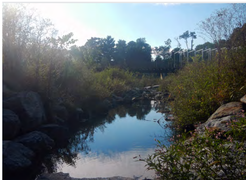
Restored stream, Evans Parkway Park Silver Spring, MD
