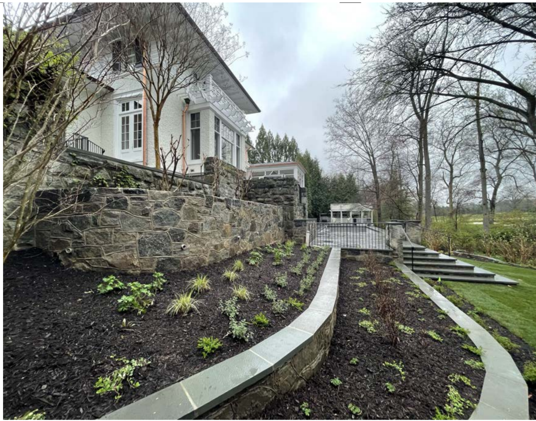
EXISTING TERRACE WALLS FROM REAR LAWN
