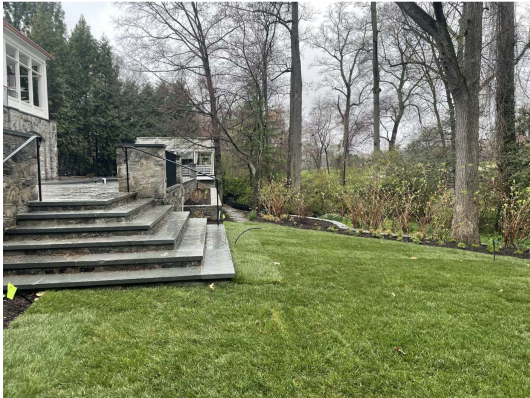
EXISTING STAIRS TO LOWER LAWN
