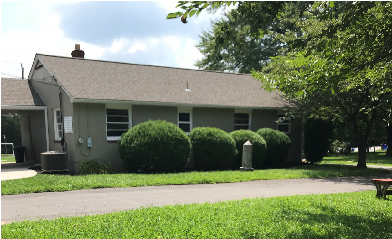
2. Approach to monument from parking lot, facing south
