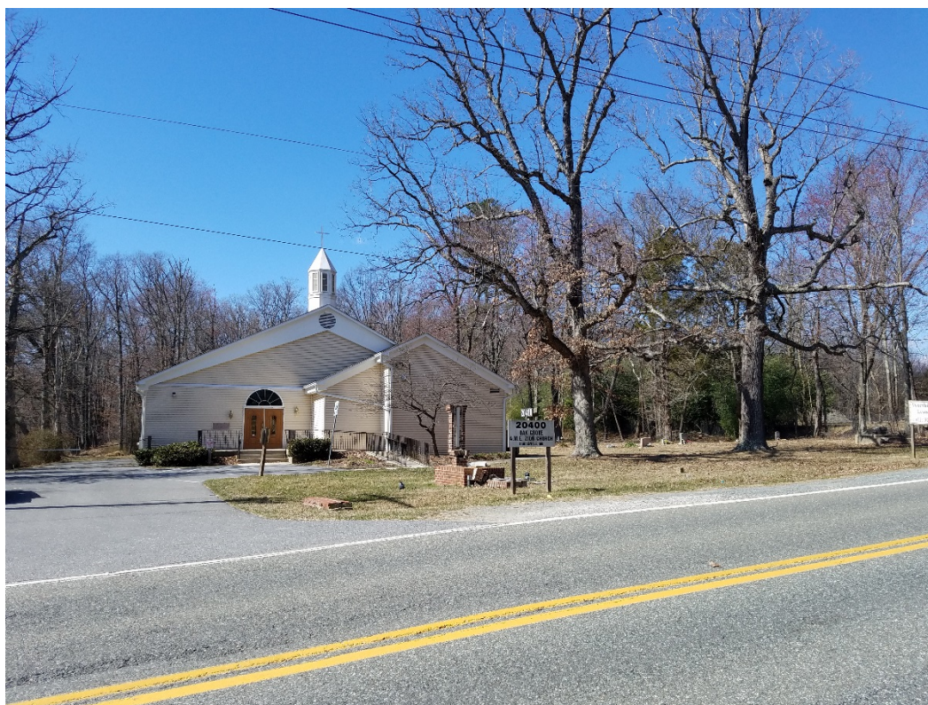
1. View of church and cemetery from Zion Road, facing northwest
