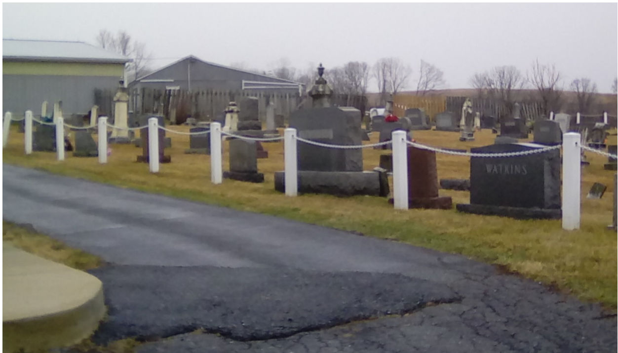
2. Access road alongside cemetery, facing west
