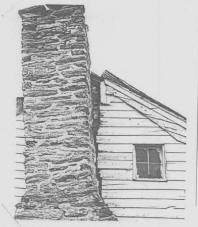
Detail of West gable end. Earlier weatherboard siding and roof line of north log Section visible to right of Chimney. March 1981
