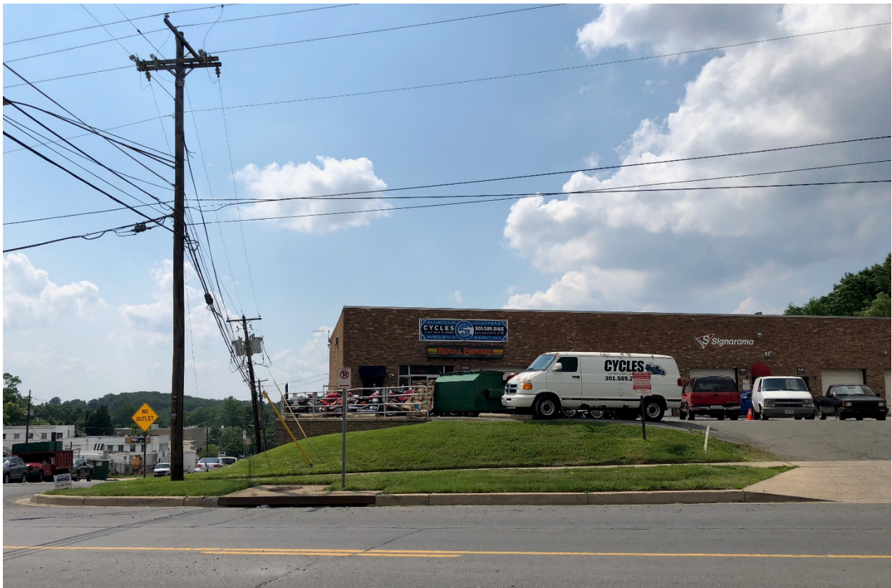
4. Currently location with industrial buildings on site
