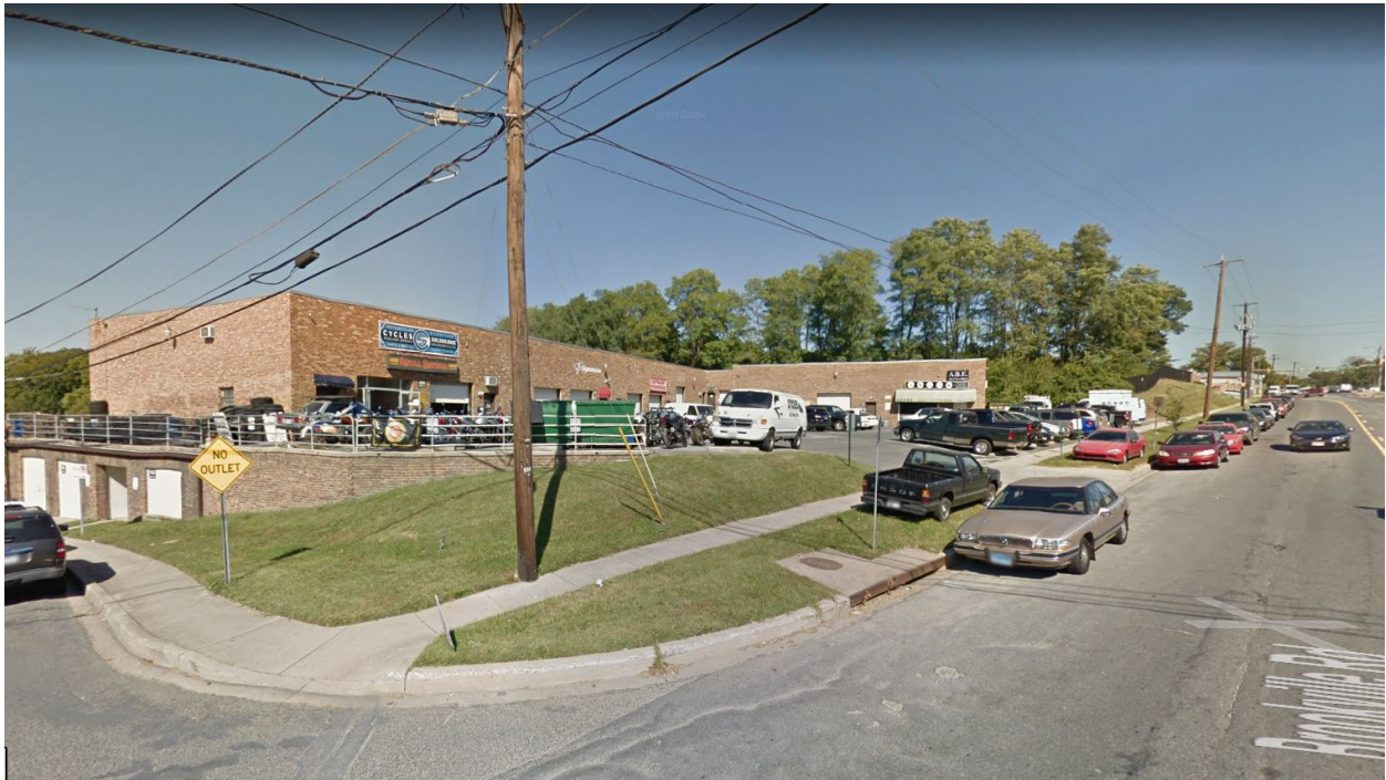
3. Currently location with industrial buildings on site
