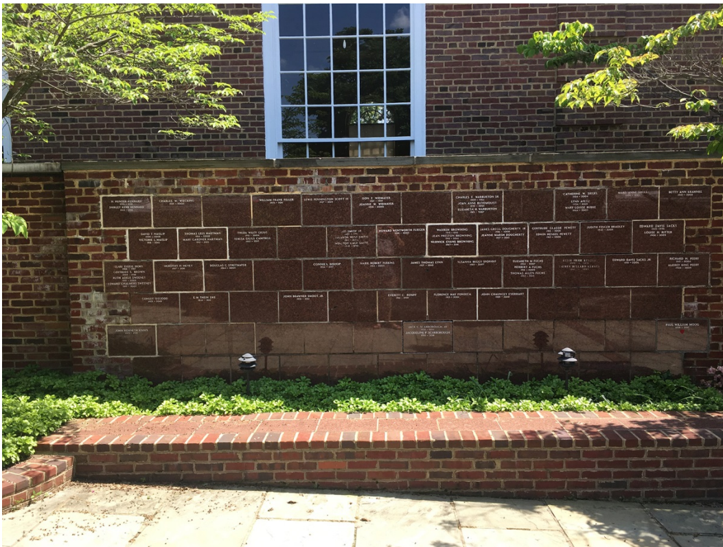
14. Vault group #3 on southern brick wall
