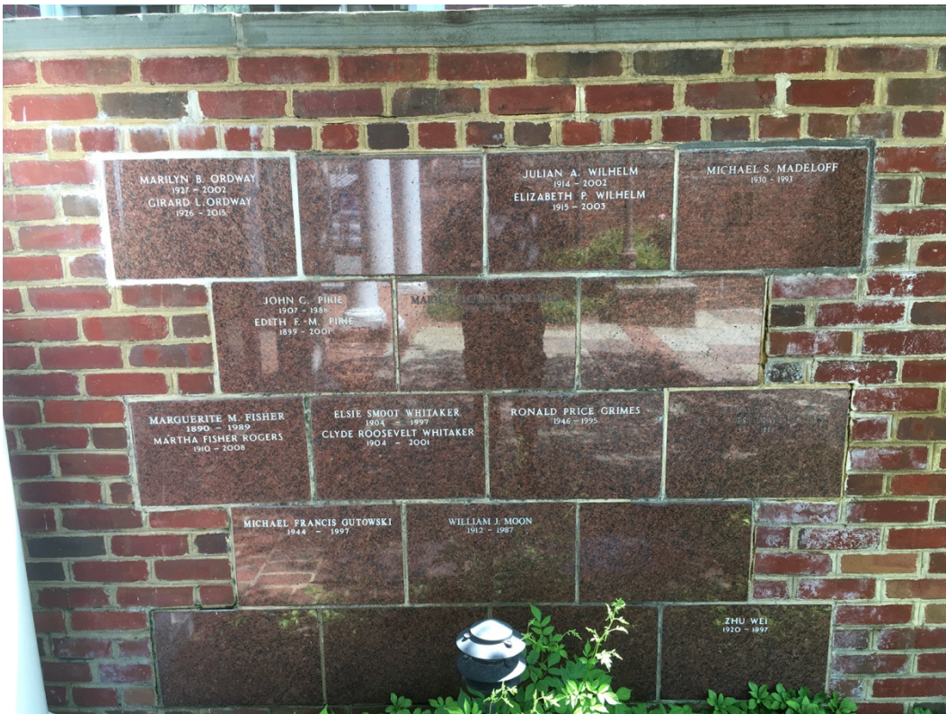
12. Vault group #1 on southern brick wall
