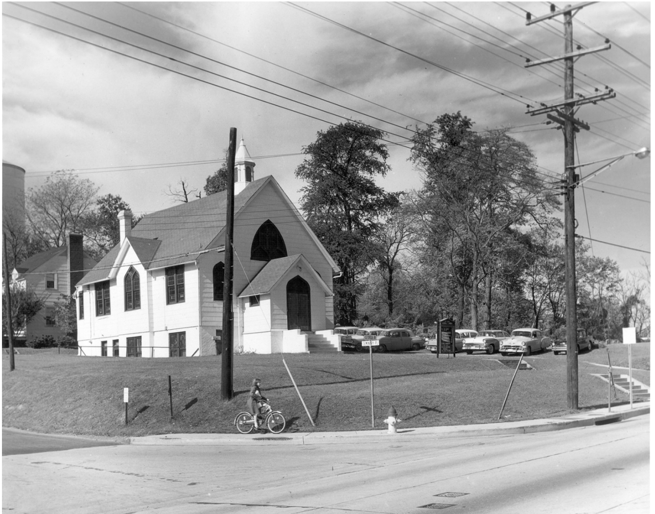
Historic photo of the church , parking lot, and cemetery behind
