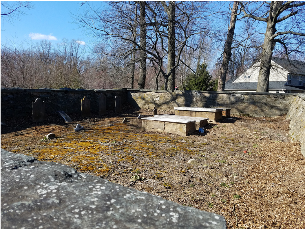
4. View to center of cemetery from southeast corner, facing north
