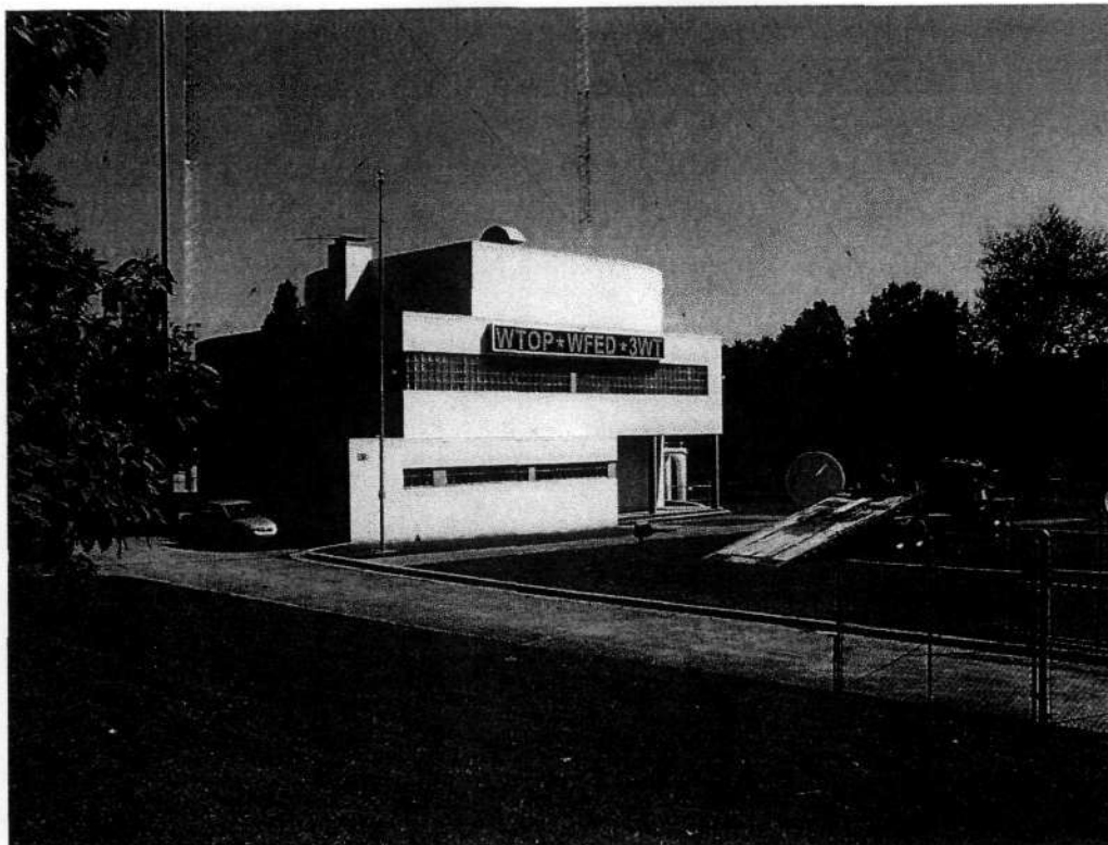
Photo 1 Looking northeast across the site.
