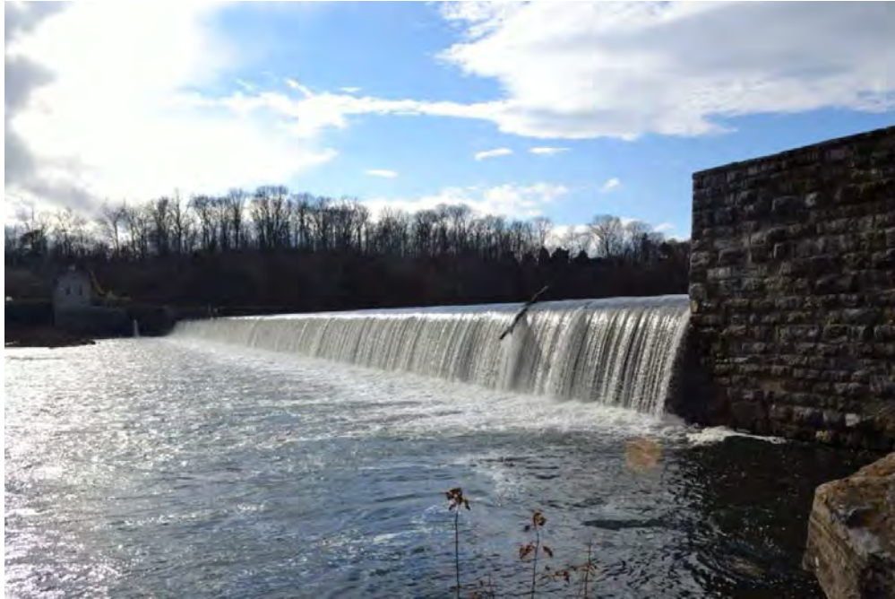
Photo #23 Mile 84.40 (Map 15). View SW to Dam 4 (00158), north of Sharpsburg, MD
