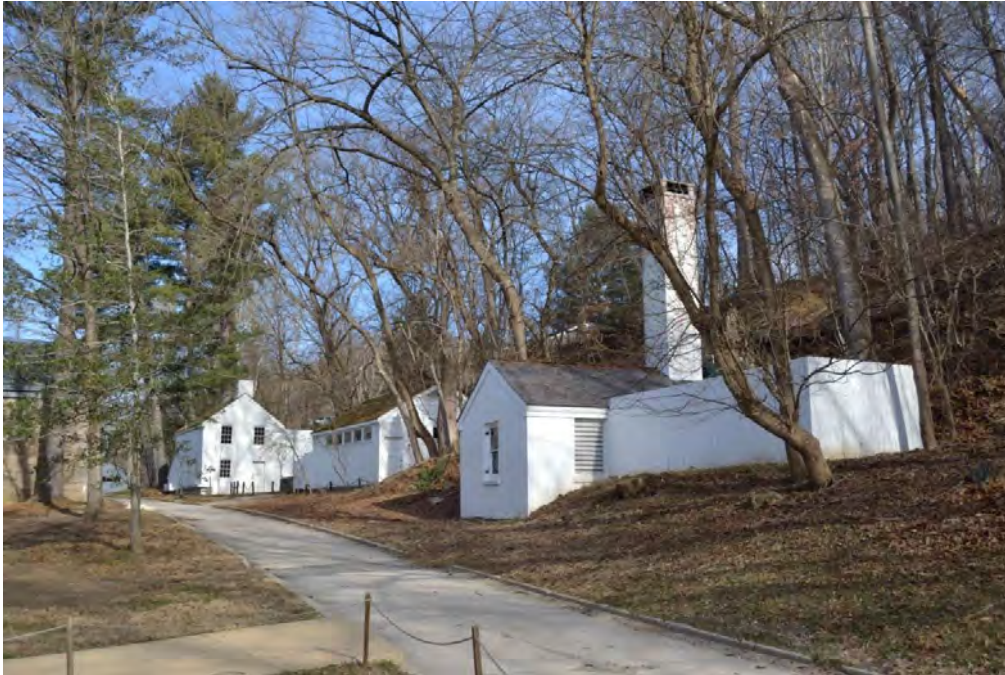
Photo #10 - Mile 14.27, 14.28, 14.29 (Map 3). View NE to Civilian Conservation Corps Buildings: Boiler House (46620), Comfort Station (46622), and Pump House (46621) at Great Falls, MD
