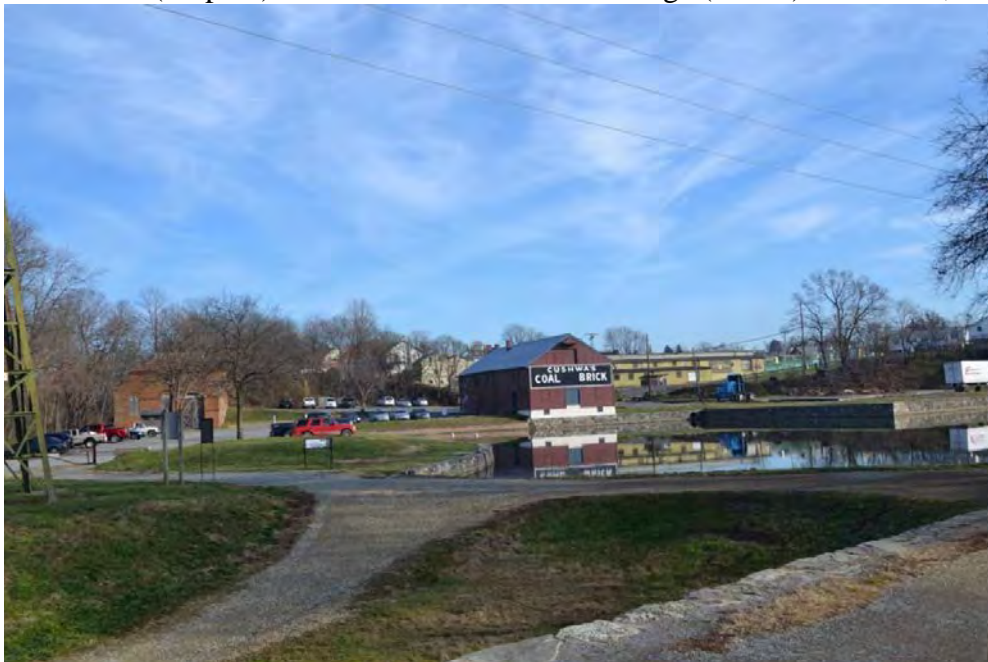
Photo #31 Mile 99.73, 99.74, 99.72 (Map 17). View ESE to Cushwa's Boat Basin (11711) in foreground, Williamsport Power Generating Station (12915) to the left, and Cushwa Warehouse (12916) in Williamsport, MD
