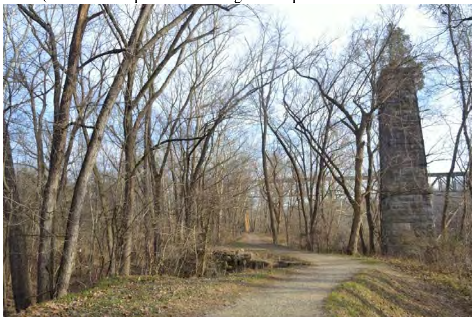
Photo #20 - Mile 72.65, 72.63B (Map 14). View SE to towpath with canal to the left, Shepherdstown River Lock (stone work left of towpath, 11701), and Shenandoah Valley Railroad Bridge Pier (right of towpath, 47512) near Shepherdstown, WV. (Railroad overpass crossing Potomac River in this image is not part of the C&O resource inventory.)
