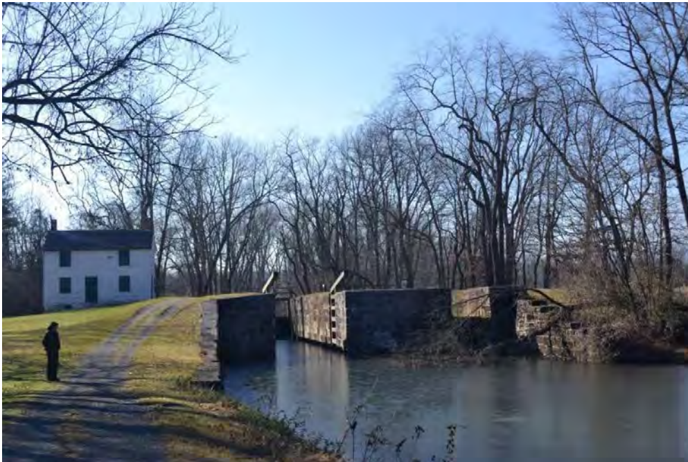
Photo #41 - Mile 175.62, 175.60, 175.61 (Map 28). View W showing Lock 75 (11771), Bypass Flume (11772), and Lockhouse – Lock 75 (11773); the last lock before the canal terminus in Cumberland, MD
