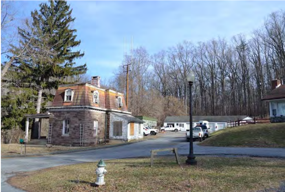
Photo #12 - Mile 14.38, 14.35 (Map 3). View E to Washington Aqueduct Gate Keeper's House with CCC-built Engineer's Garage (no LCS#) in background and a non-contributing 1956 engineer's house to the right at Great Falls, MD
