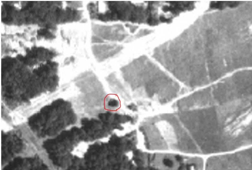
1970 Aerial (during development excavation)
