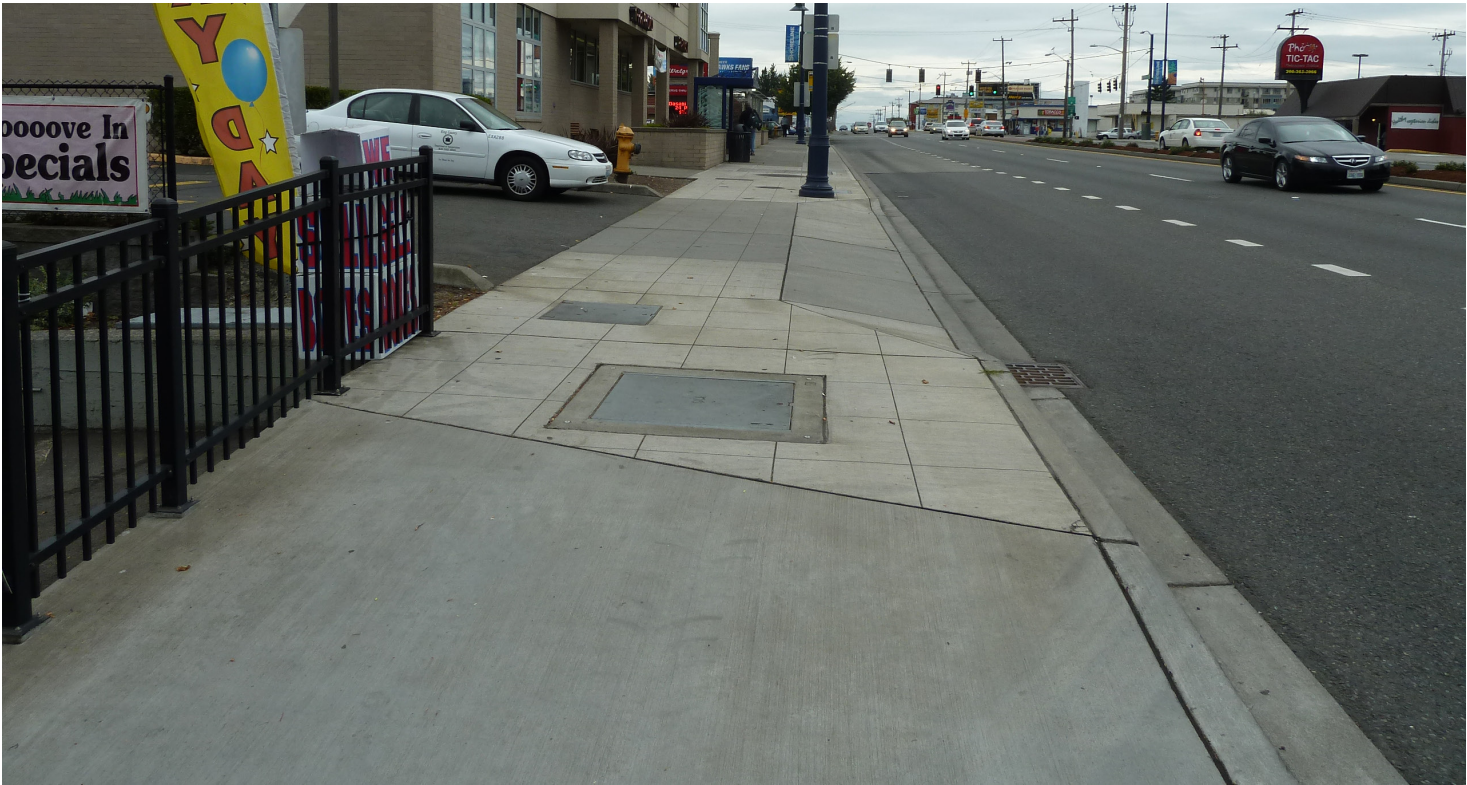
FIGURE 24 Driveway with sidewalk continuing across driveway opening
