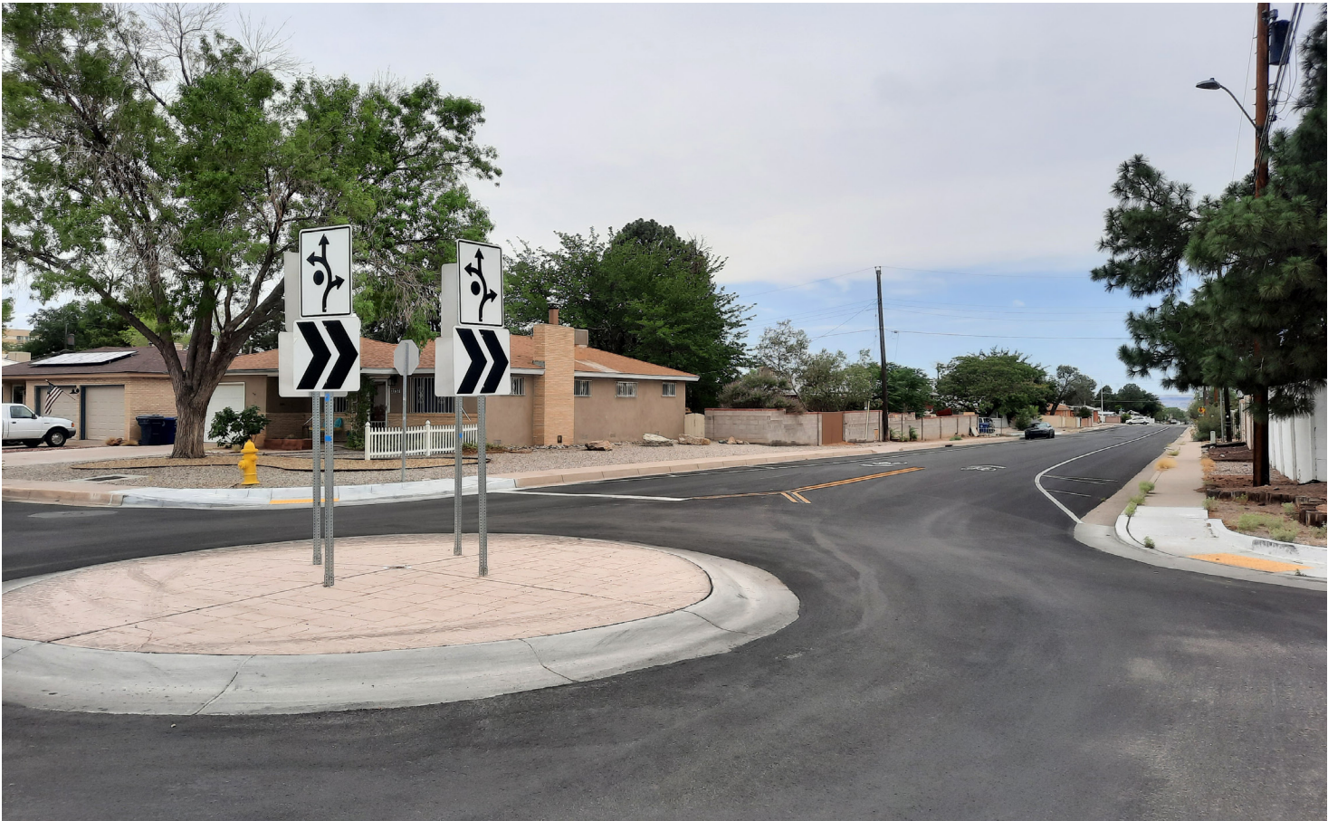
FIGURE 38 Roundabout with a mountable center island
