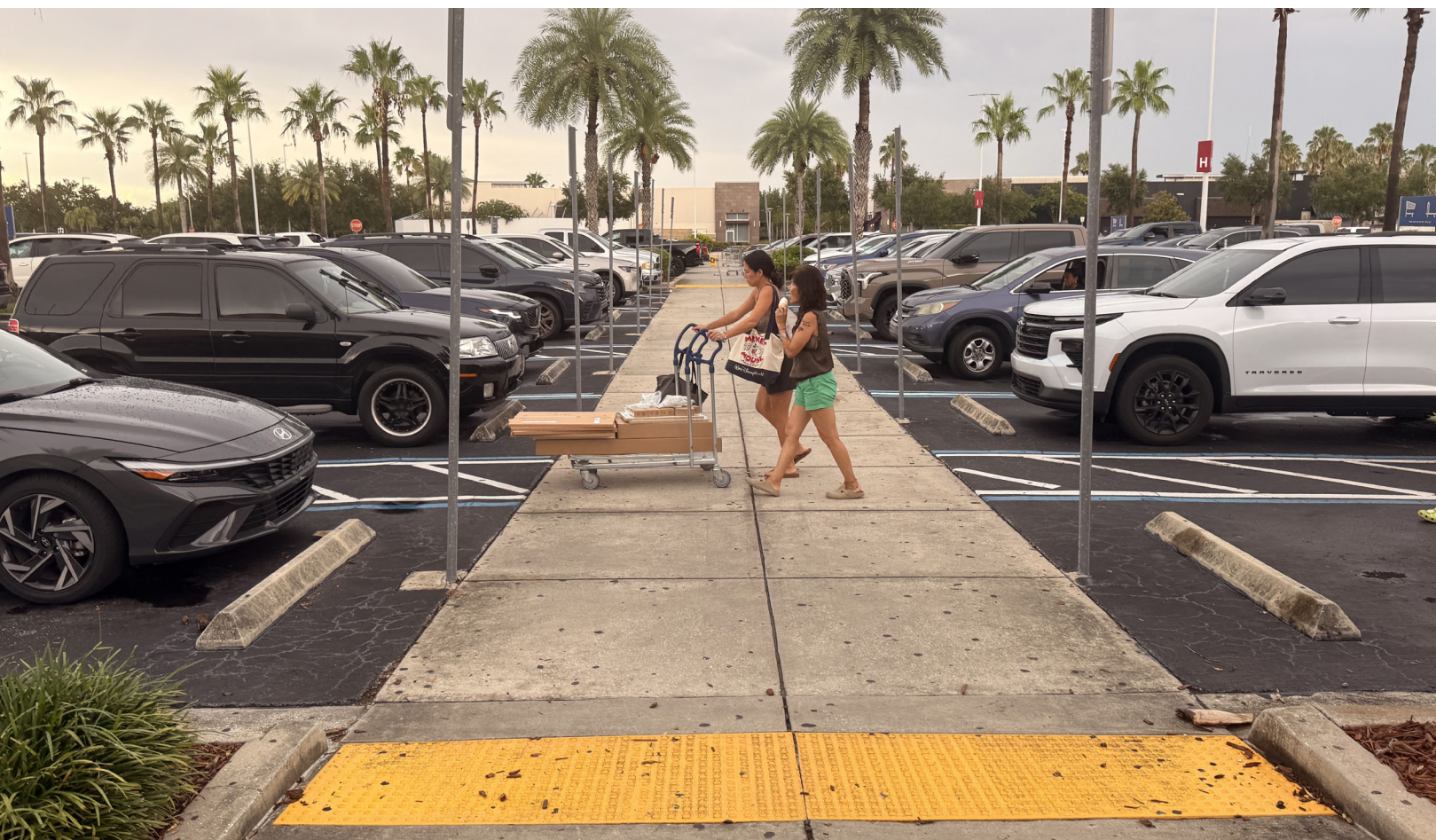
FIGURE 15 Street-level centerwalk protected by wheelstops
