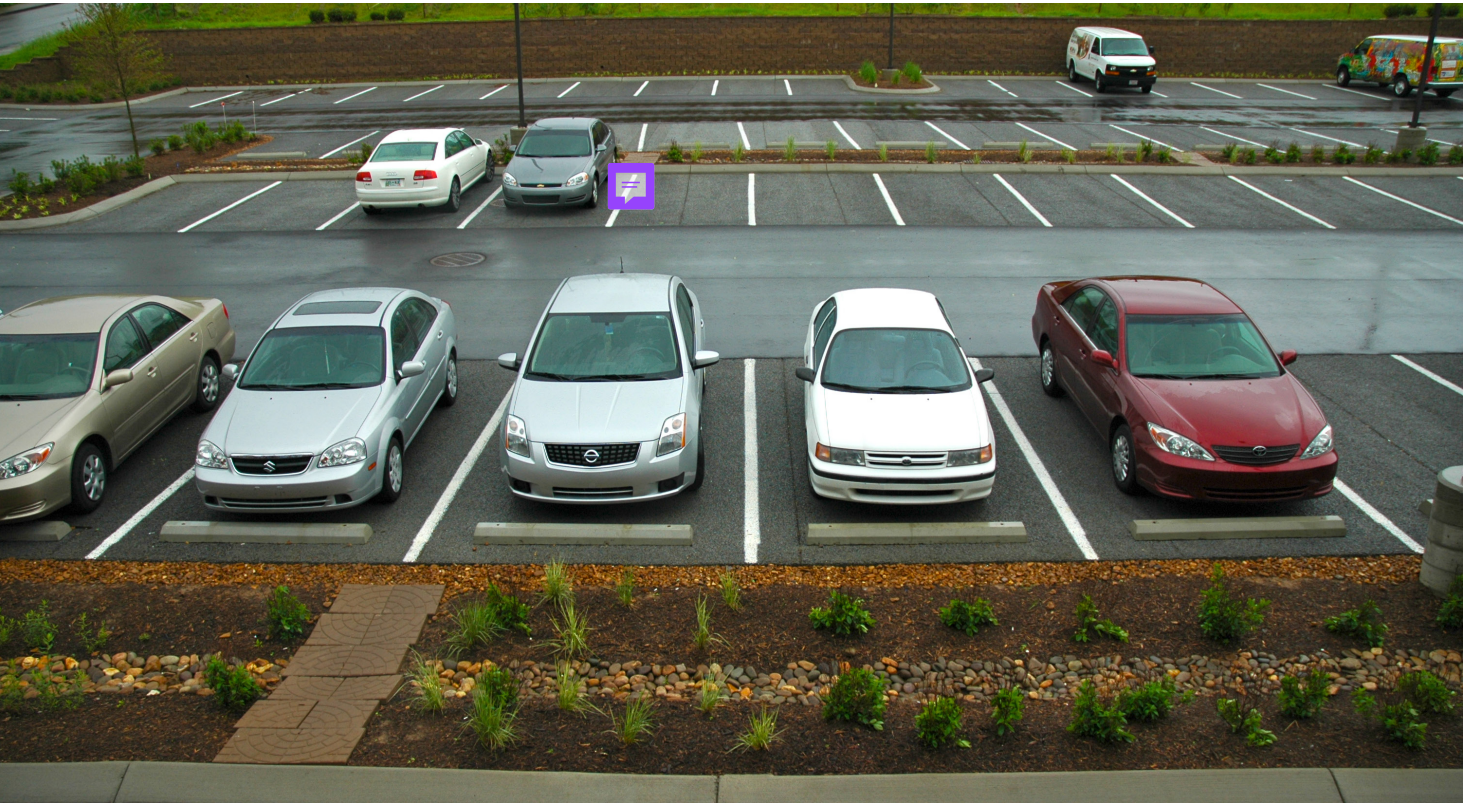
FIGURE 37 Stormwater management on end islands
