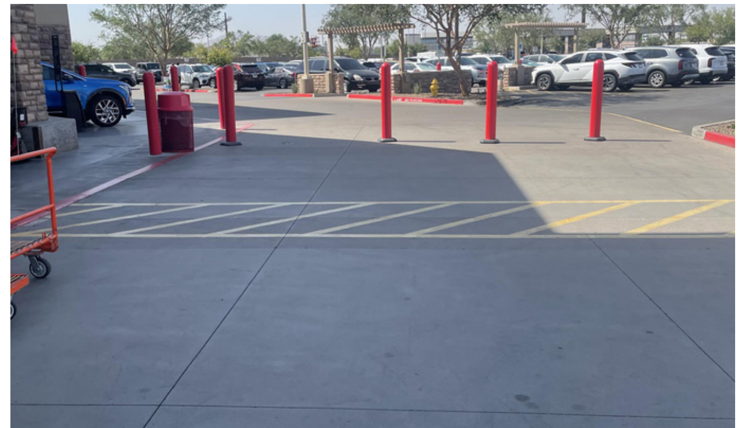
FIGURE 7 Building frontage road (BFR) terminated with bollards
