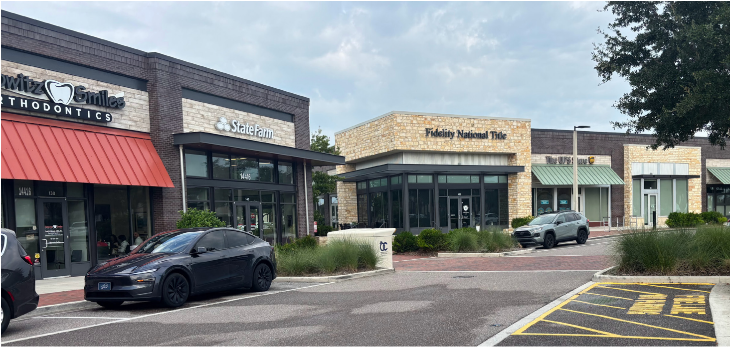
FIGURE 28 Curb extensions in a parking lot
