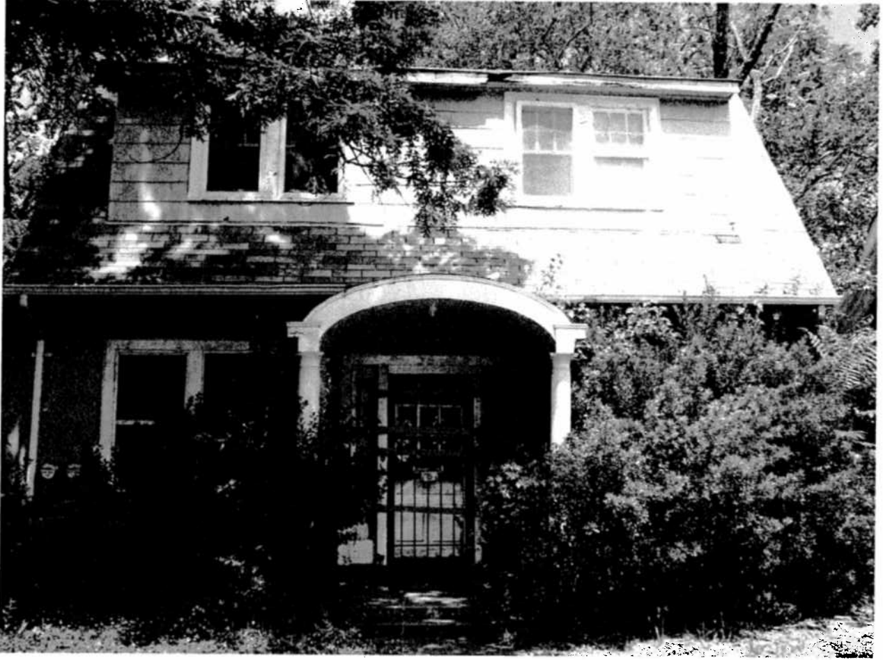
36 PHILADELPHIA AVENUE, TAKOMA PARK MD – SW / FRONT ELEVATION
