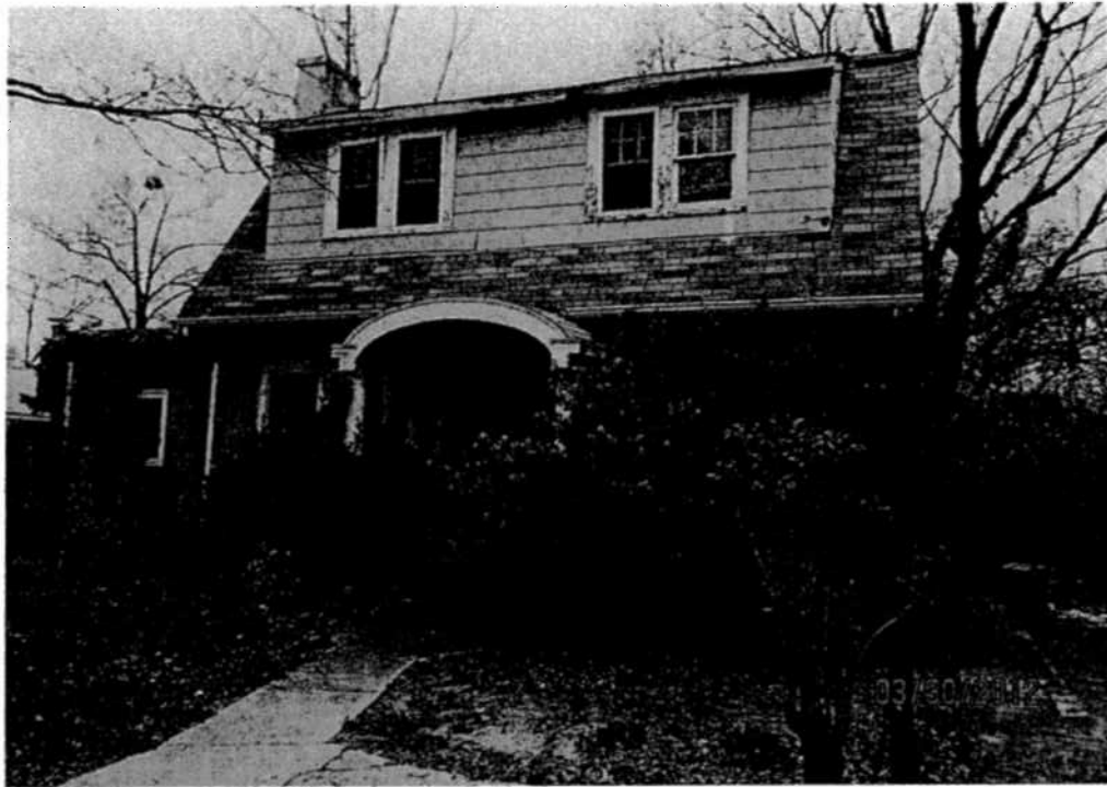
1. General front view of 36 Philadelphia Ave.
