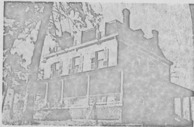
NO. 110 E-9 ADRIAN R. WADSWORTH 1853-54 STONE RUBBLE FILLED WITH CEMENT MORTAR
