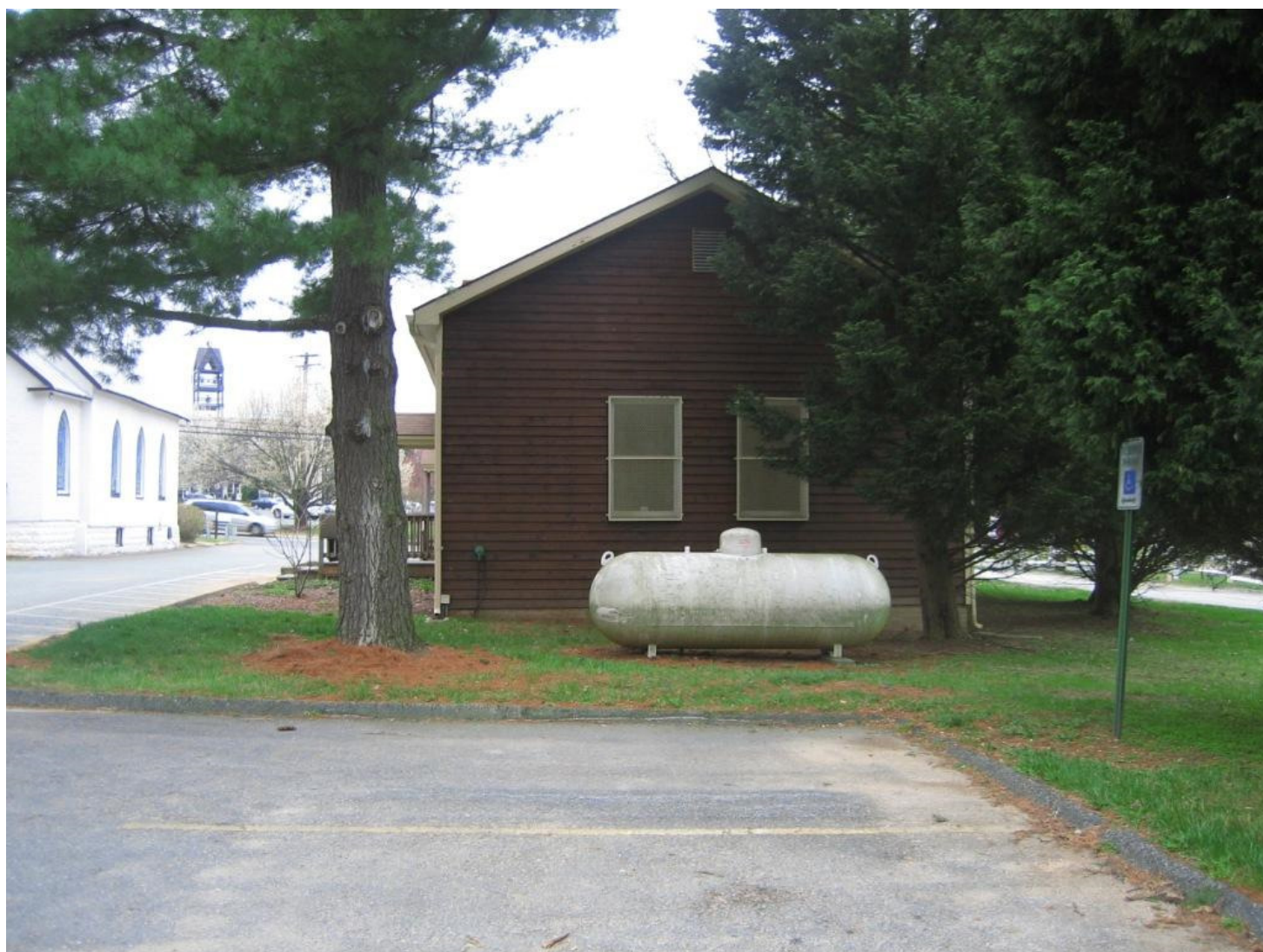
Figure 12. View of Norbeck Recreation Center, north elevation.
