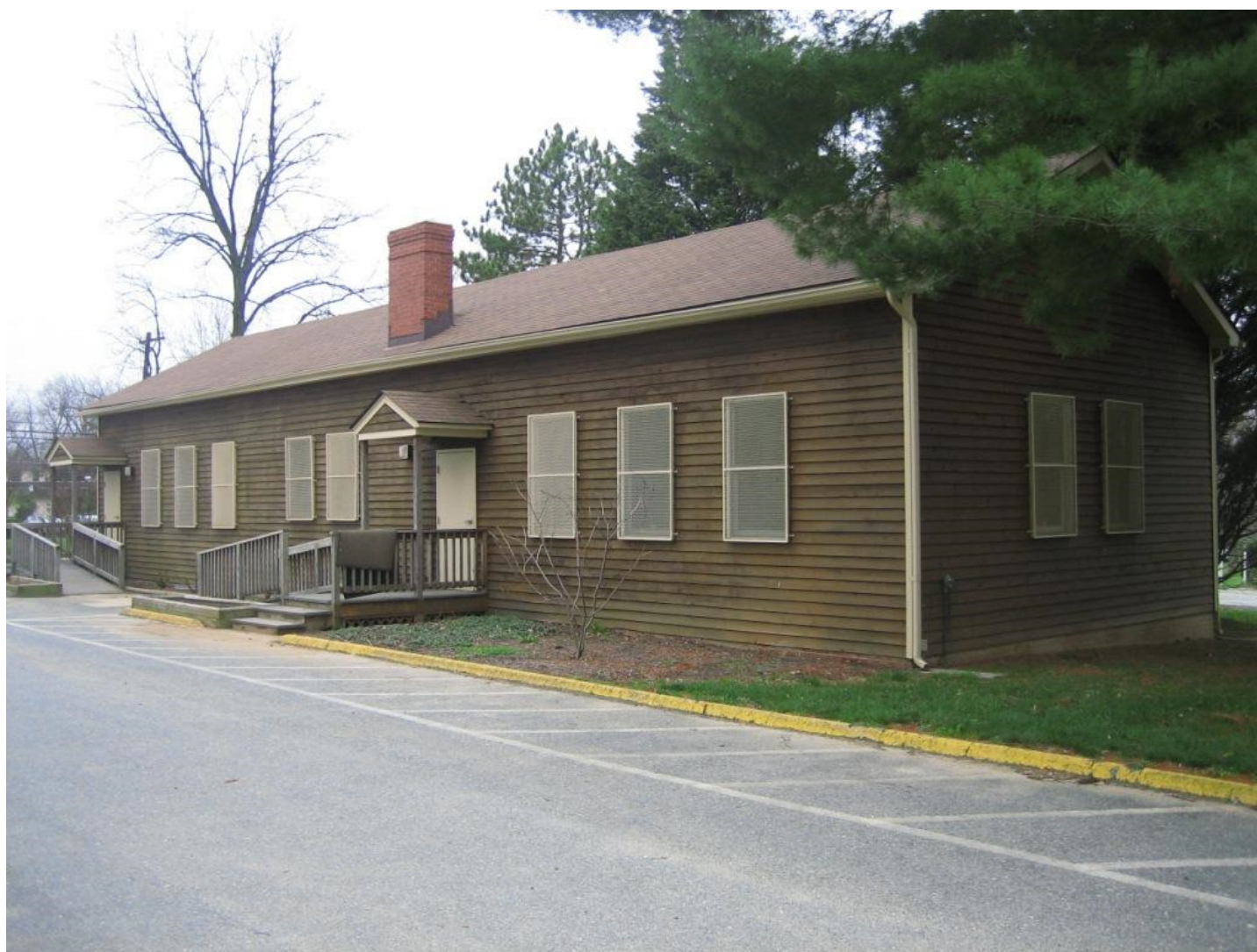
Figure 11. View of Norbeck Recreation Building, northeast corner.
