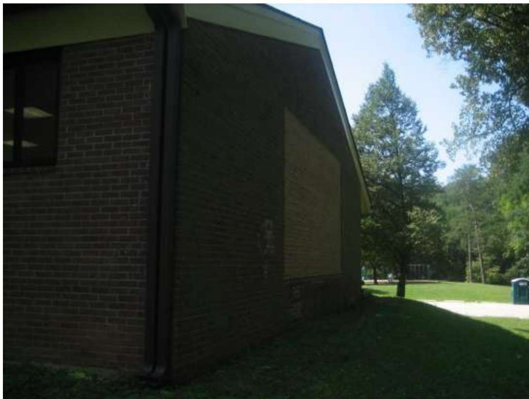
Figure 13. View of Veirs Mill Recreation Building, south elevation.
