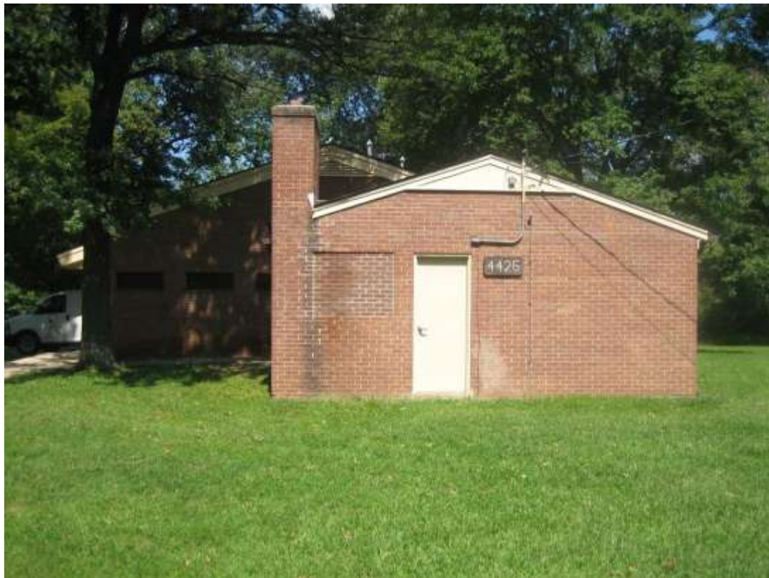
Figure 10. View of Veirs Mill Recreation Building, north elevation.
