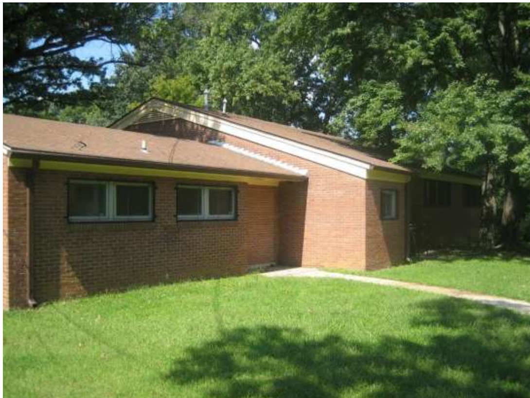
Figure 11. View of Veirs Mill Recreation Building, west (rear) elevation.
