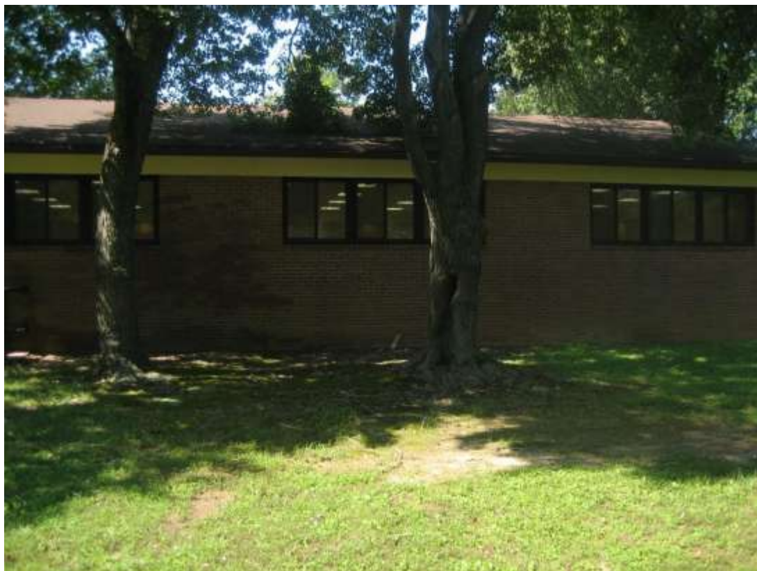
Figure 12. View of Veirs Mill Recreation building, west (rear) elevation.
