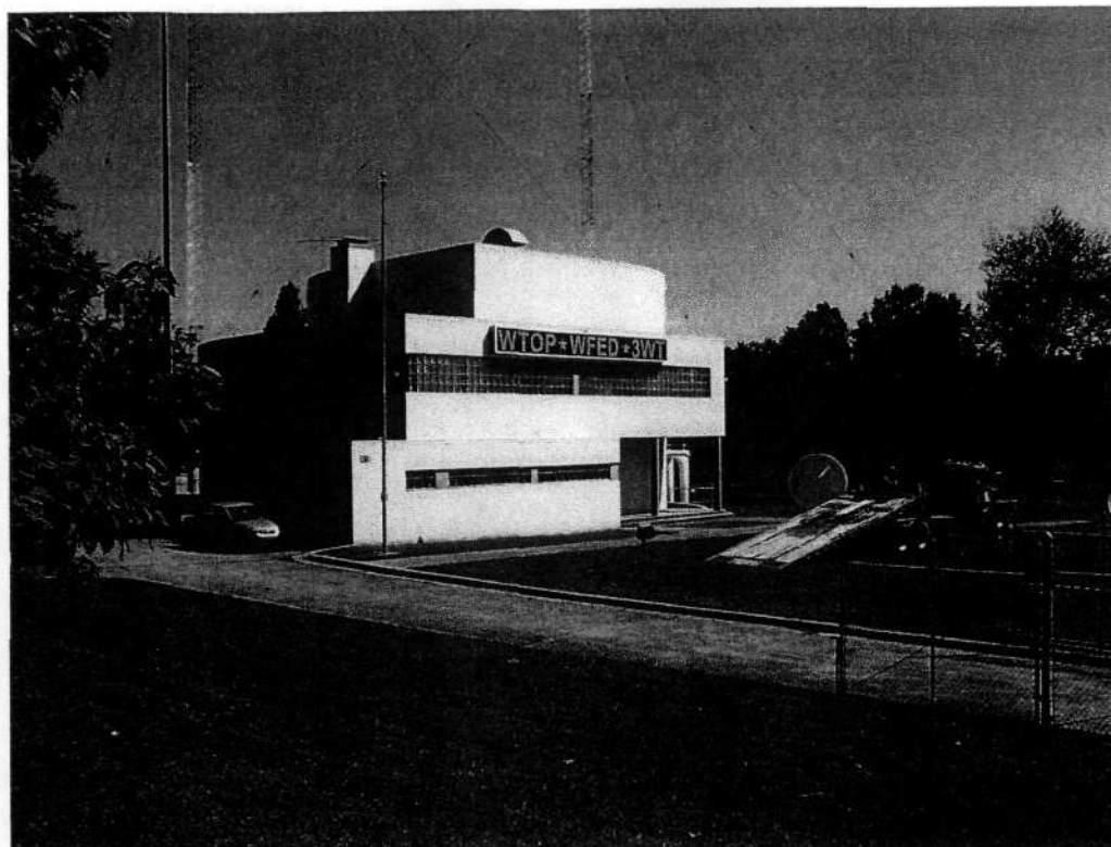
Photo 1 Looking northeast across the site.
