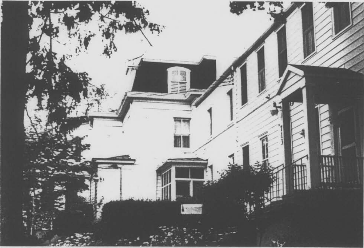
Rear facade of mansard roofed block (center) with mid-20th century addition at right. Photographer: Joyce DeLaurentis, M-NCPPC, 5-1998.
