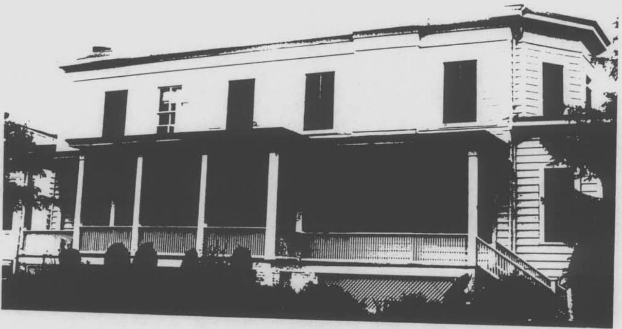
Current view of front elevation.
