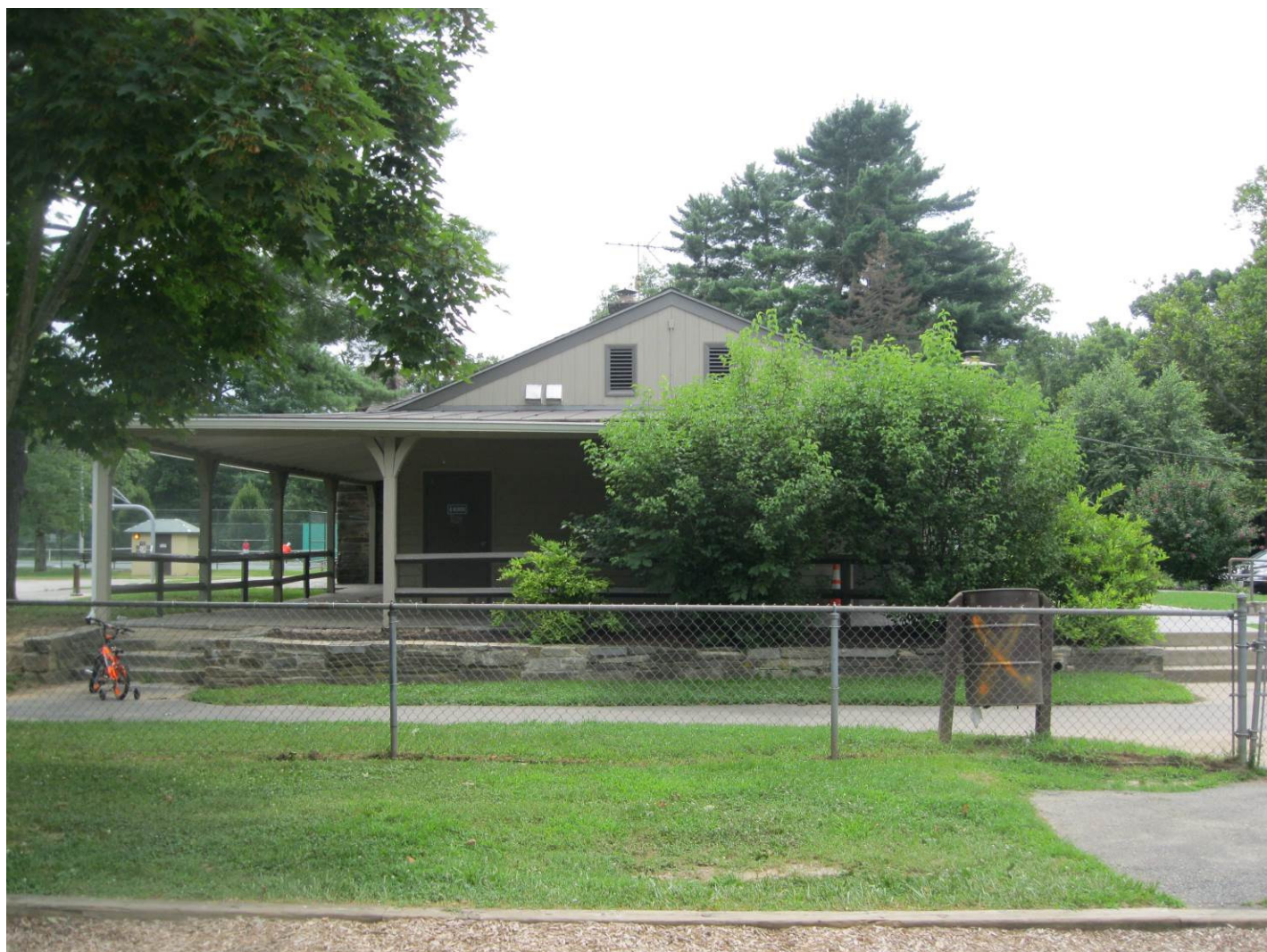
Figure 19. View of Meadowbrook Recreation Building, from playground; north elevation.
