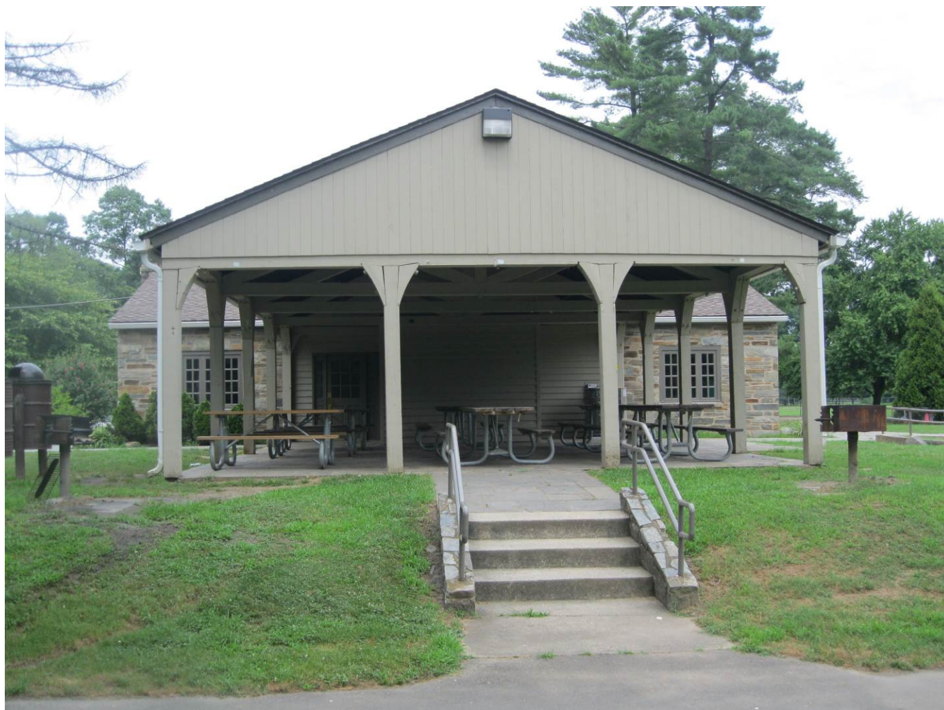
Figure 15. View of Meadowbrook Recreation Building, south elevation.
