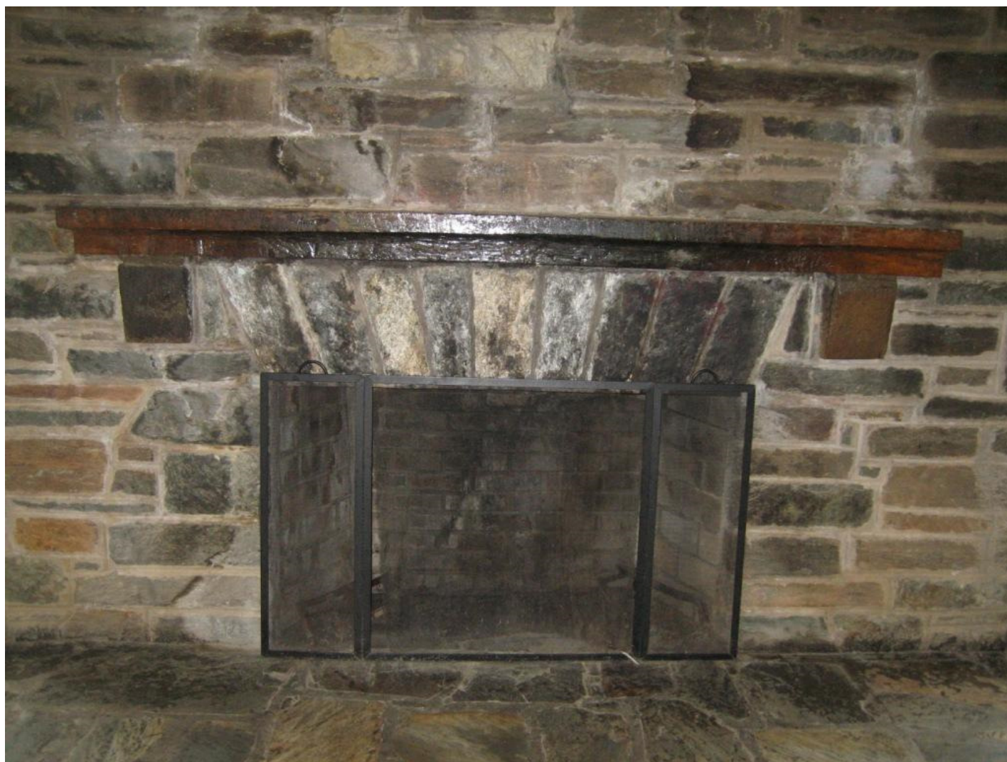
Figure 23. Detail of interior hearth, fireplace, and mantel, Meadowbrook Recreation Building.
