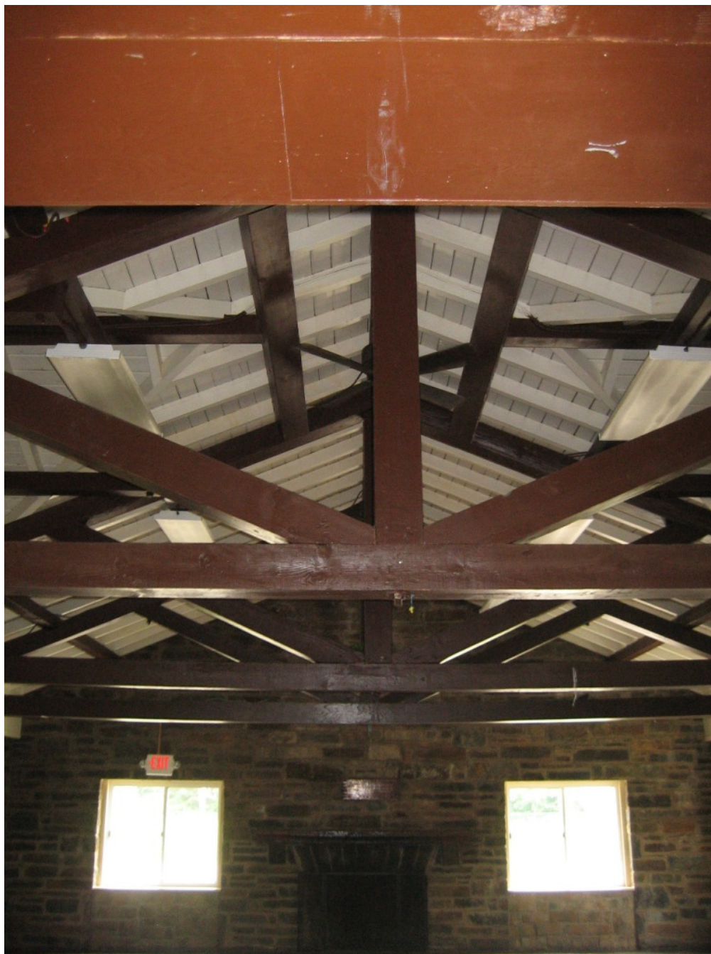
Figure 24. Detail of exposed, rough-hewn trusses at interior ceiling, Meadowbrook Recreation Building.
