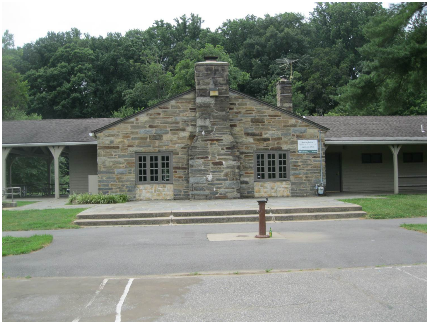
Figure 17. View of Meadowbrook Recreation Building, west (rear) façade.
