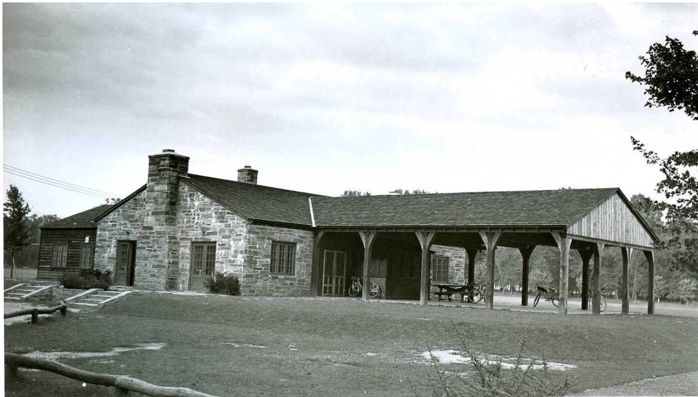
Figure 9. Rock Creek Recreation Center, c1940s. Courtesy: M-NCPPC.
