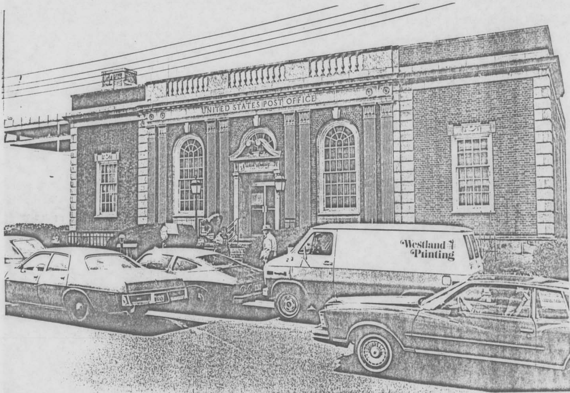
Silver Spring, Maryland, Main Post Office, front (east) elevation
