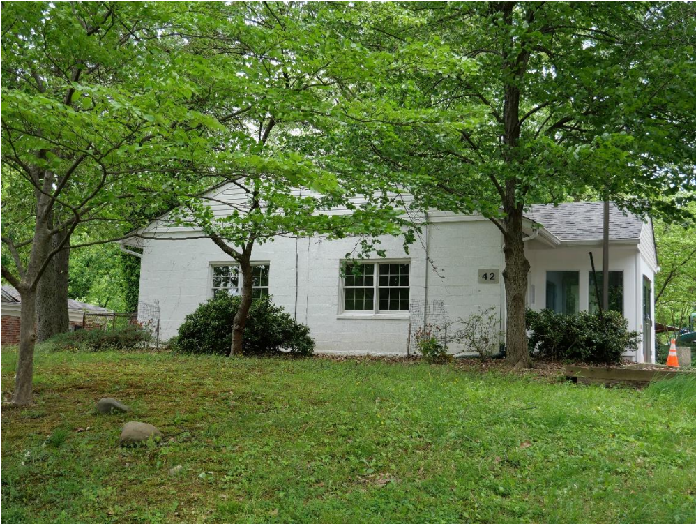
Figure 6: View of the east elevation.
