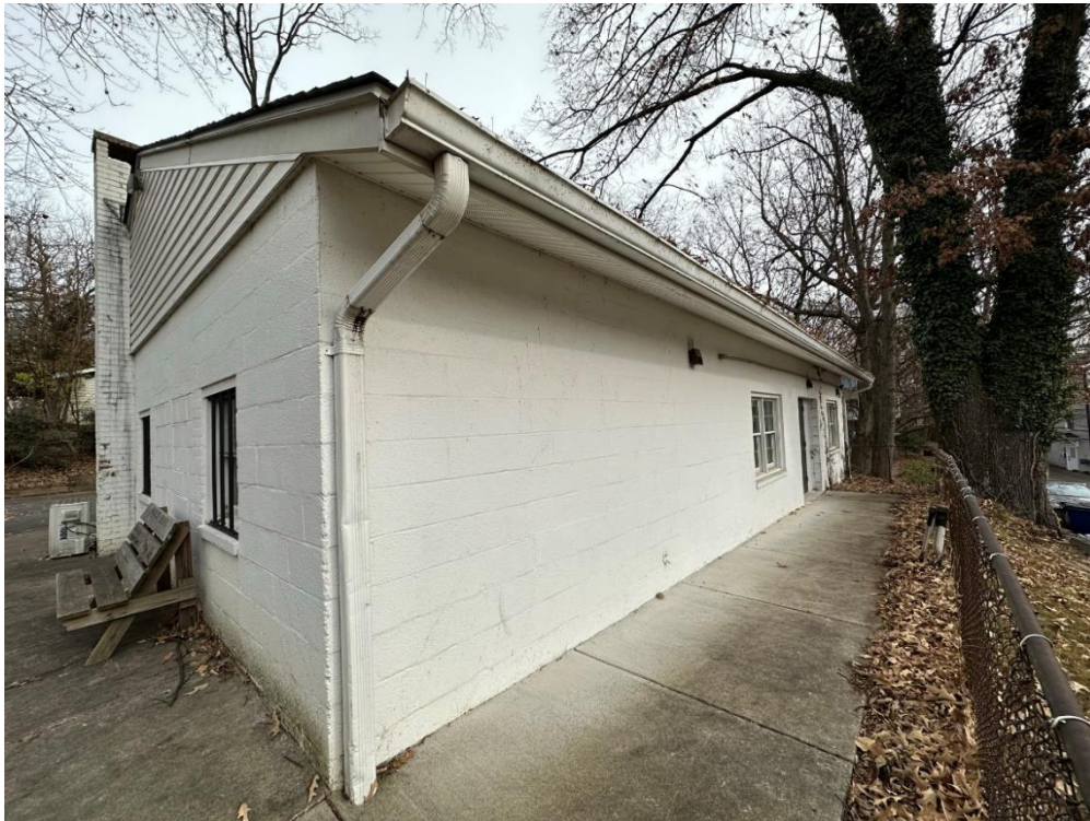
Figure 4: View of the southwest corner.
