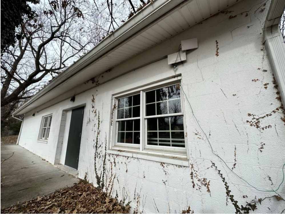
Figure 5: View of the south elevation (rear) from the southeast corner.
