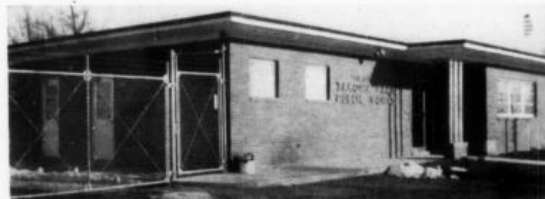
All public works business in Takoma Park is now conducted in this modern, well equipped administration building.
