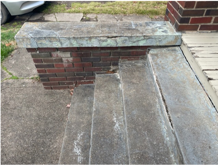
inside face of north wall
