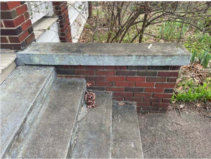
inside face of south wall
