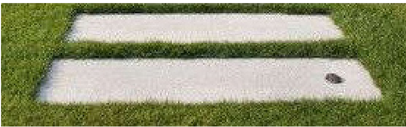
large format pavers (36" x 18"), material and finish to be selected by owner
