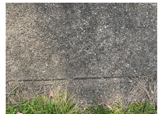
existing exposed aggregate finish
