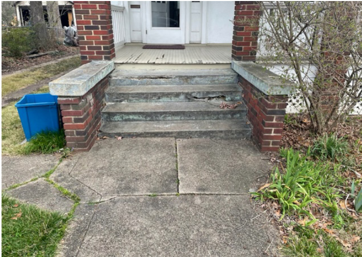
stairs and wingwalls
