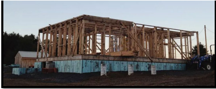
(1) It starts with the Foundation and Framing
