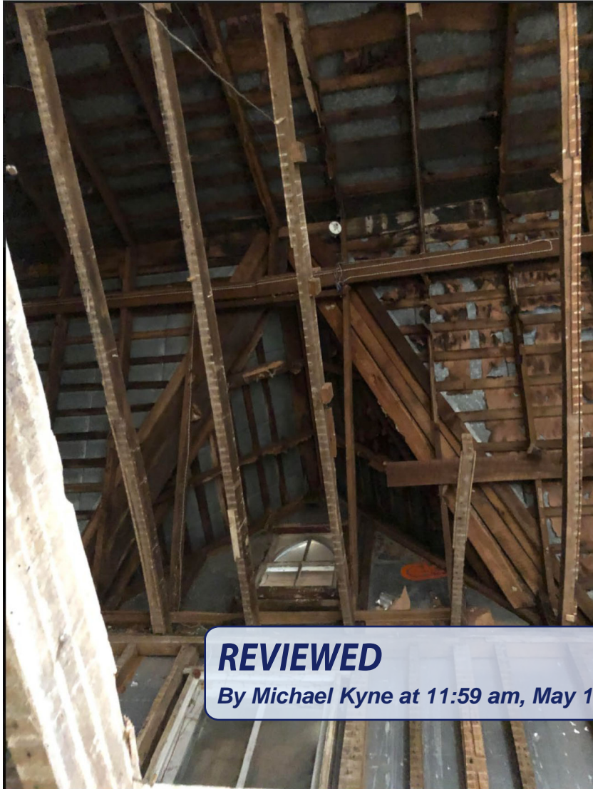
Interior Main Gable and Front Dormer
