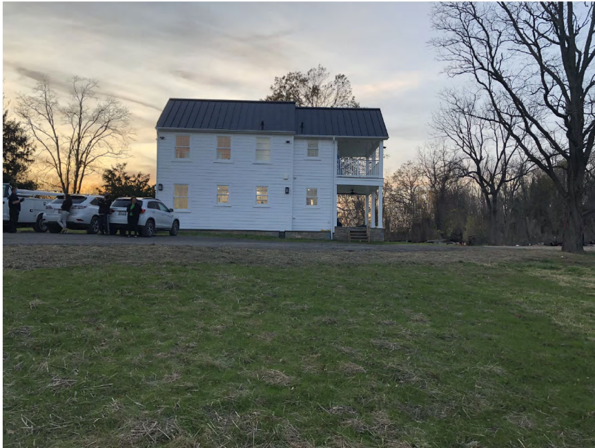
VIEW OF EAST ELEVATION OF MAIN HOUSE (NEW BARN LOCATED TO RIGHT BEYOND PHOTO FRAME)
