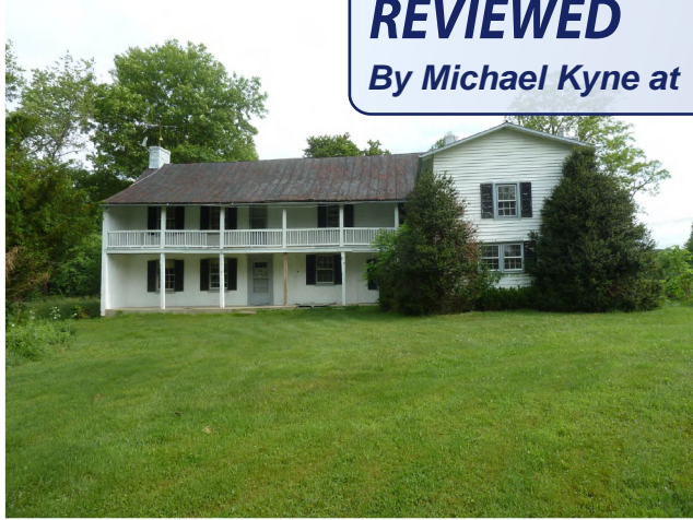
SOUTH ELEVATION VIEW BEFORE RESTORATION, 2015
