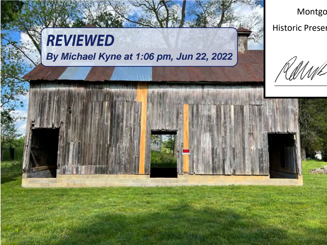
Figure 2. East Elevation: Three Open Barn Doorways; Proof-of-concept siding patching
