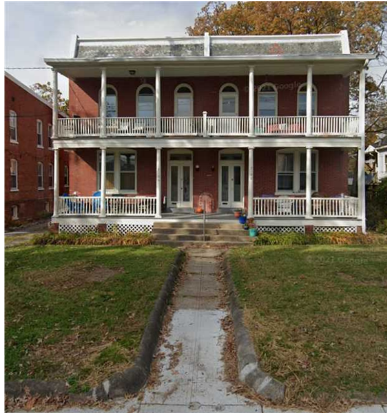
2 Street View of Building A01
