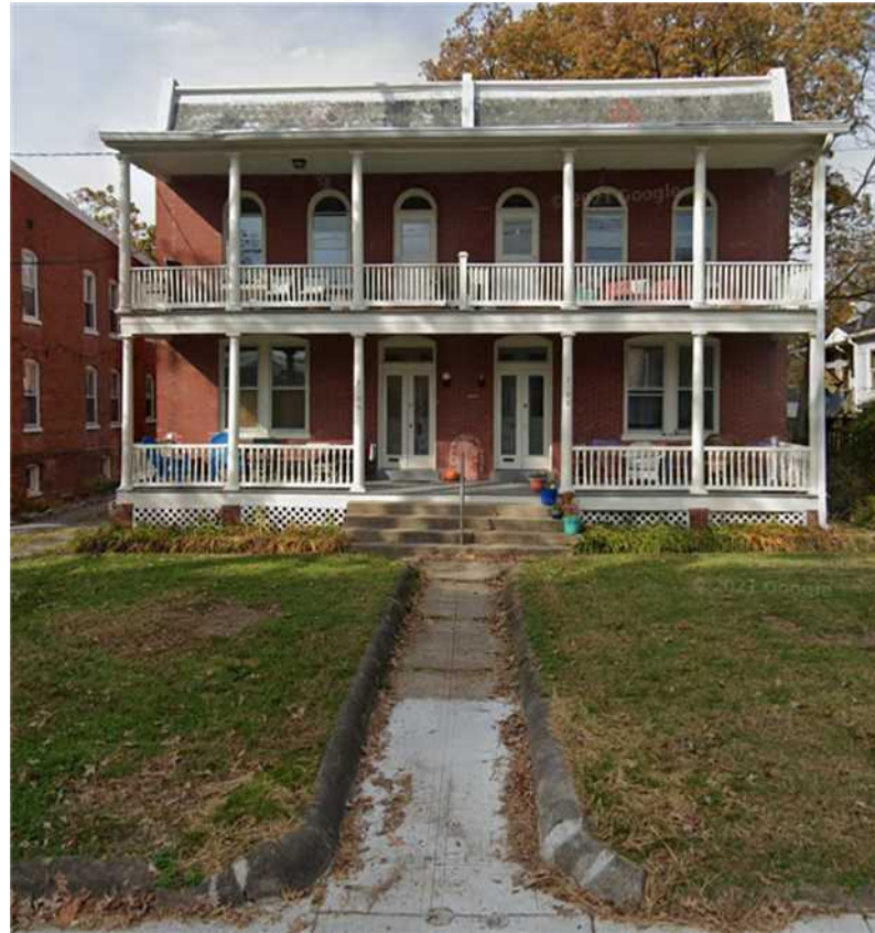
2 Street View of Building A01
