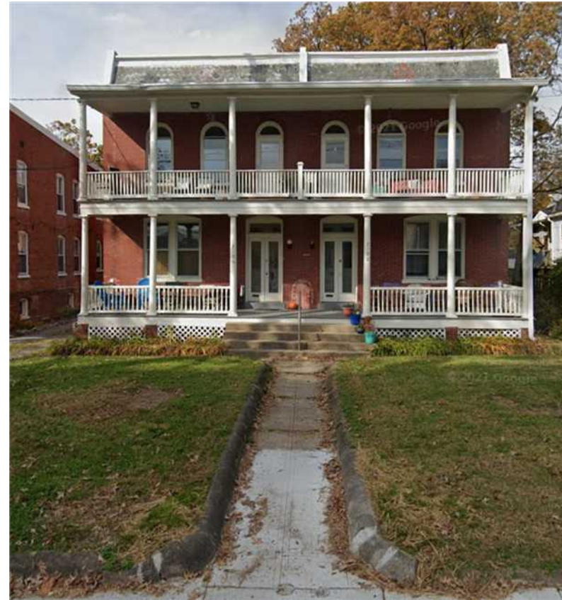
2 Street View of Building A01
