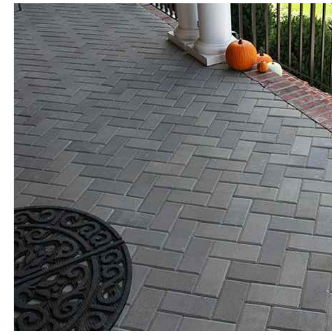
Pavers in Herringbone Pattern at Driveway w/ Chamfer Edge
