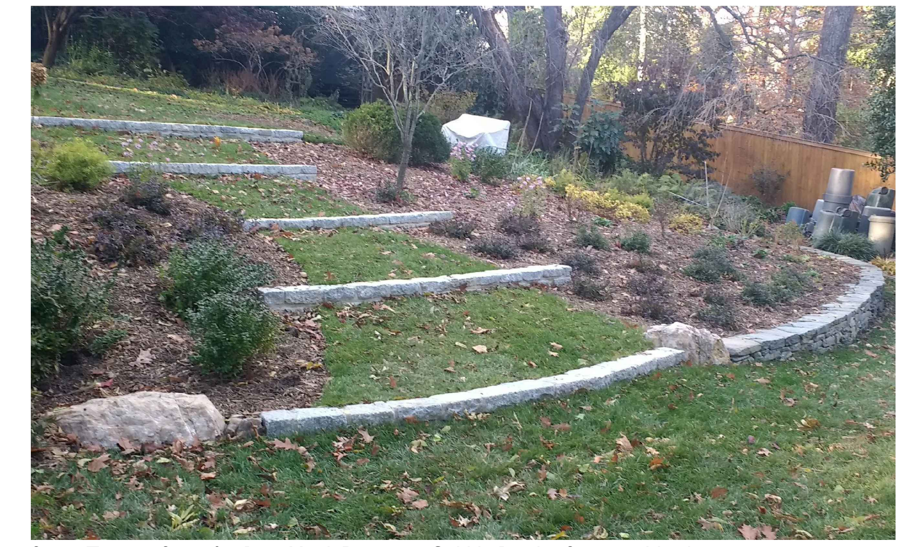
Stone Terrace Steps for Rear Yard, Driveway Cobble Border Stone to Match
