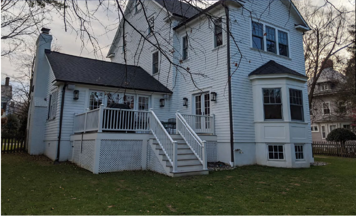
1 11 E. LENOX STREET AREA OF WORK, NORTH ELEVATION A702 NOT TO SCALE
