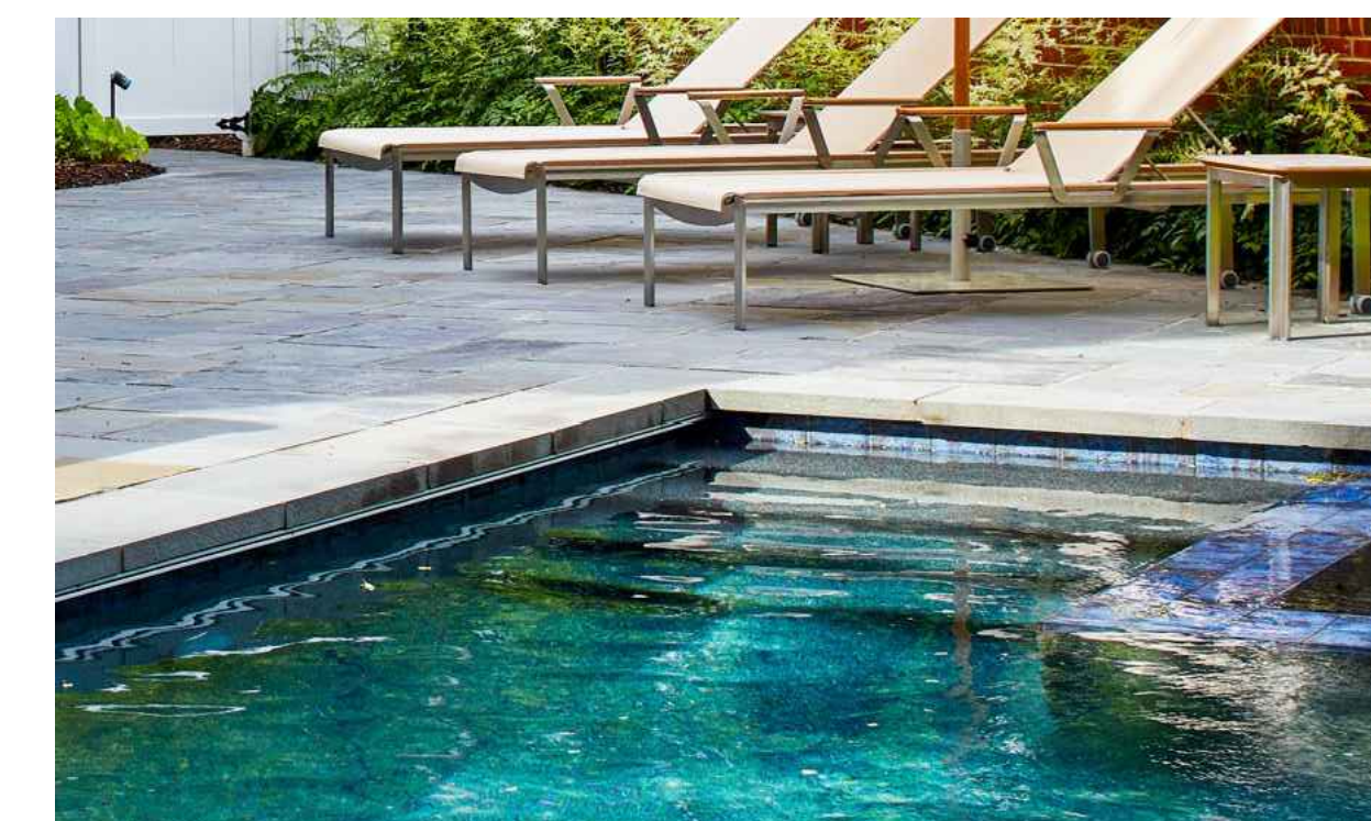
POOL COPING EXAMPLE (THERMAL BLUESTONE)
