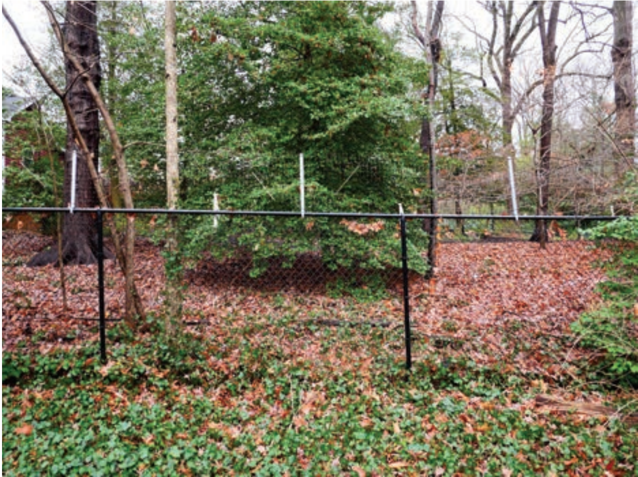
Chain-link fence with extenders along north property line with 7407 Baltimore Ave.
