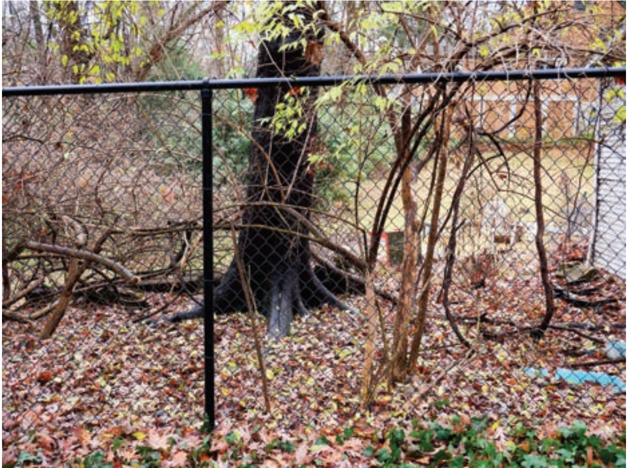
Chain-link fence in rear yard.
