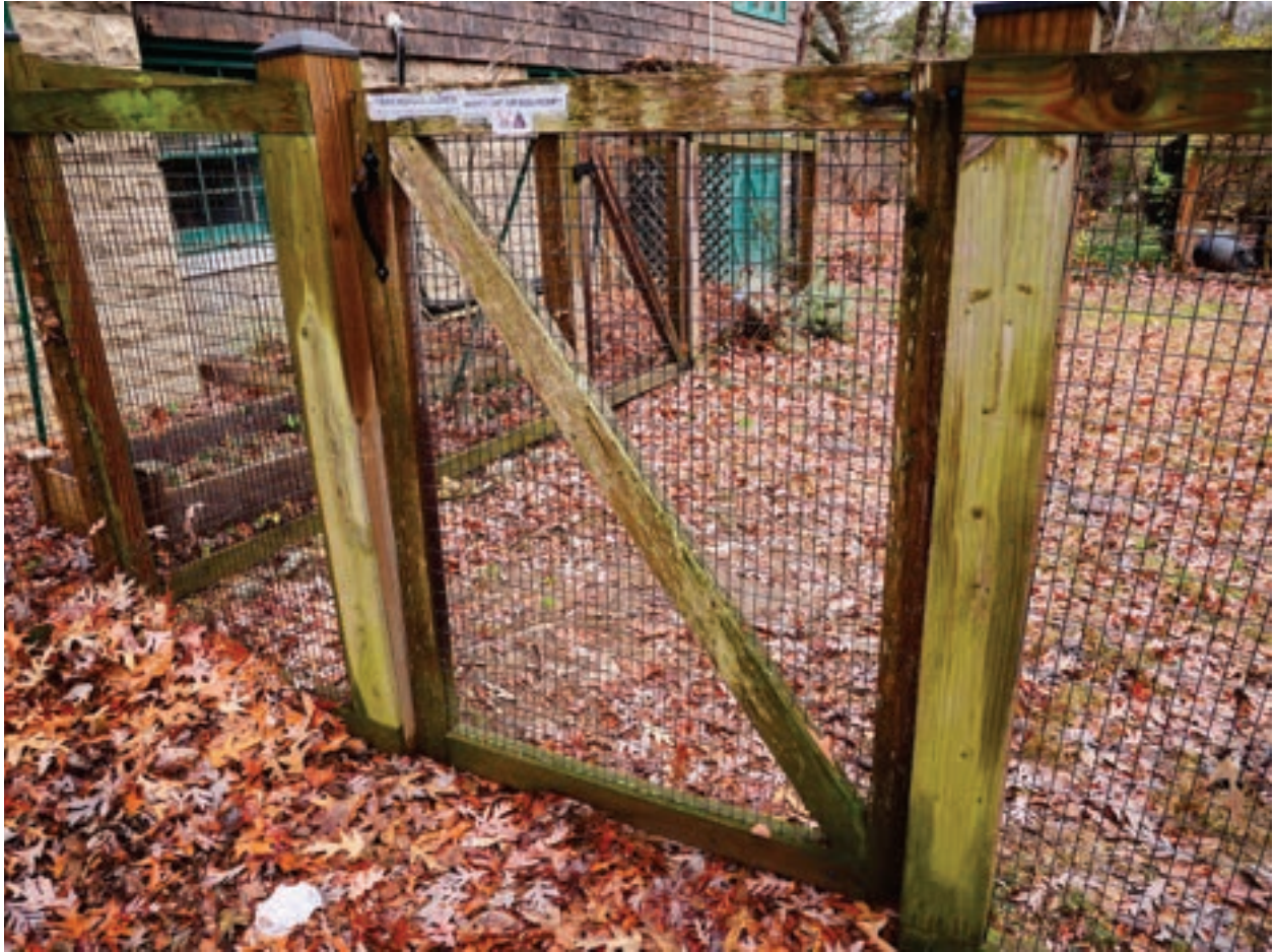
Wood and wire fence in side yard.
