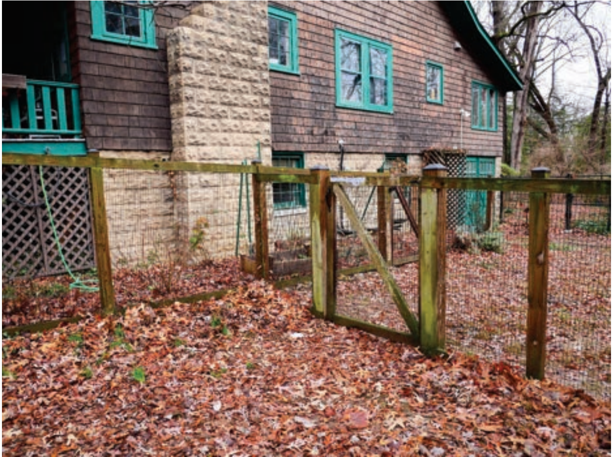
Wood and wire fence in side yard
