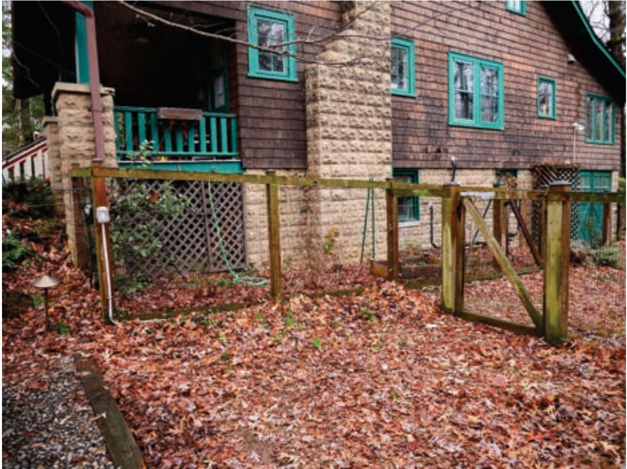
Wood and wire fence in side yard.
