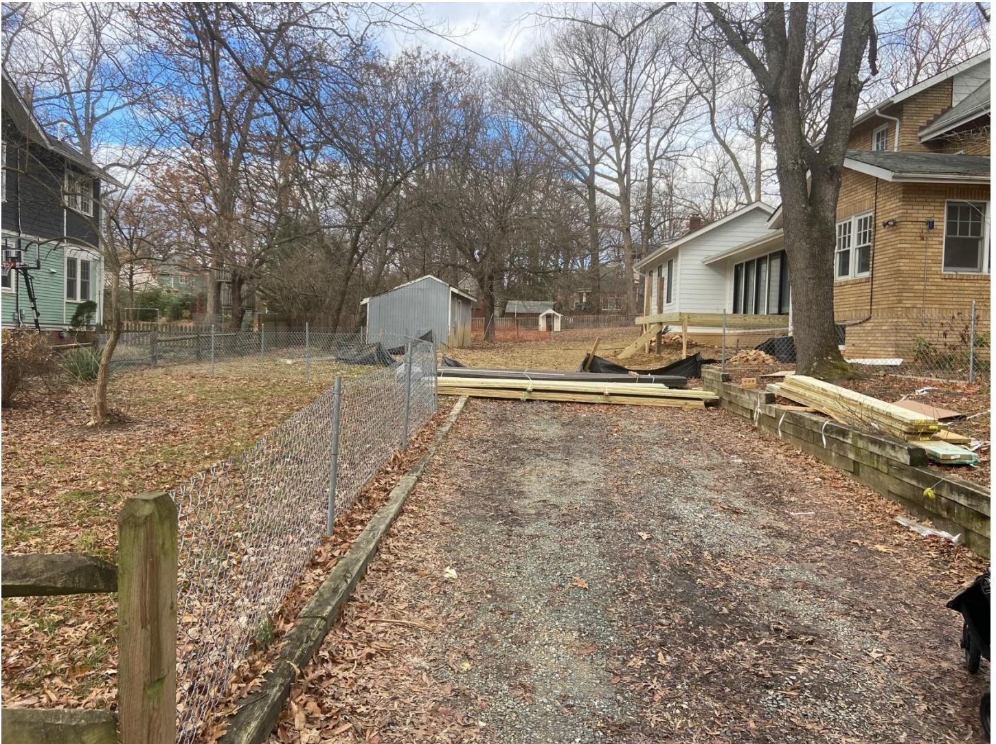
View of the accessory shed structure from the sidewalk along Takoma Ave at driveway.
