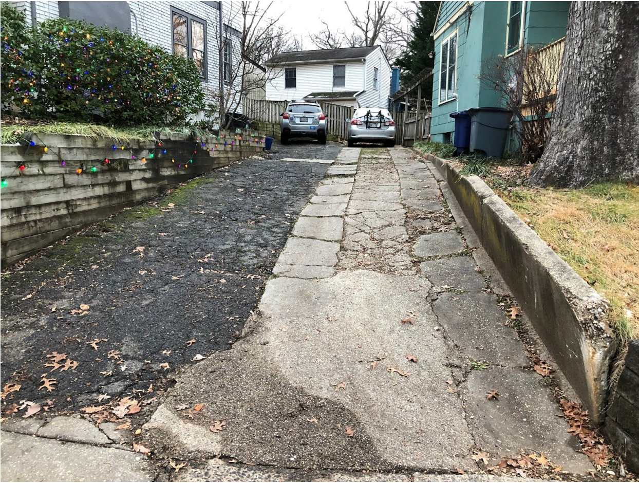
Driveway and left side retaining wall
