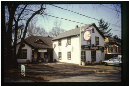
Pre-existing Conditions 1990s
