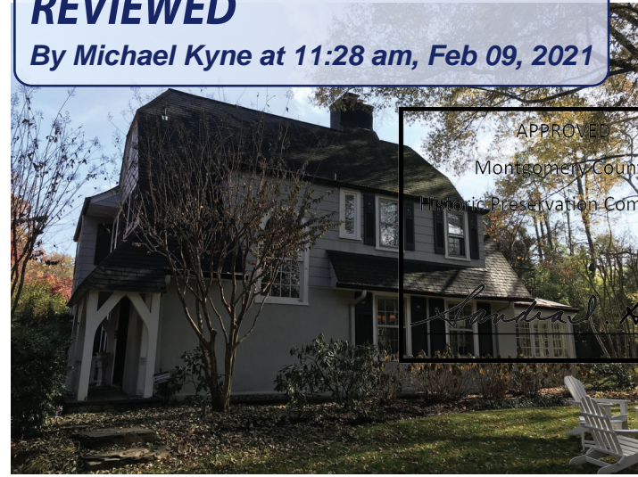
View of Side from Cedar Parkway
