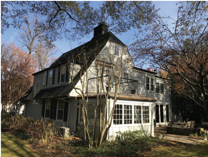
View of Rear from Cedar Parkway
