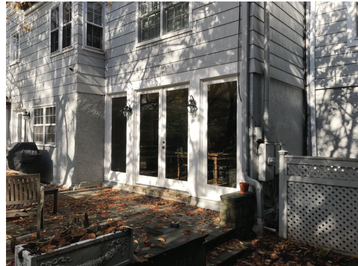
View of Rear Entry
