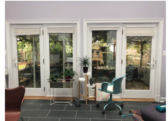
EXTERIOR DOORS BETWEEN SUNROOM AND MASONRY DECK
