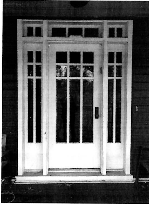
Detail: Existing Library Door (original front door), no existing storm door
