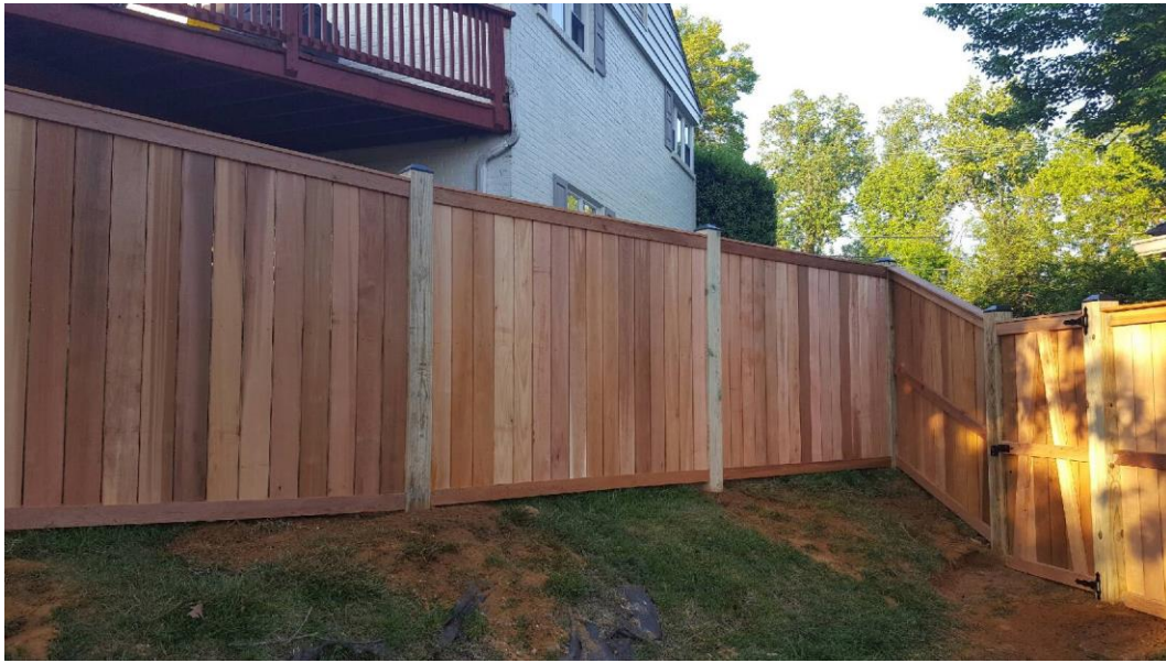
Example of Flat Board Fence
