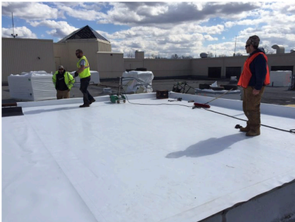
In-progress photo of a TPO roof installation
