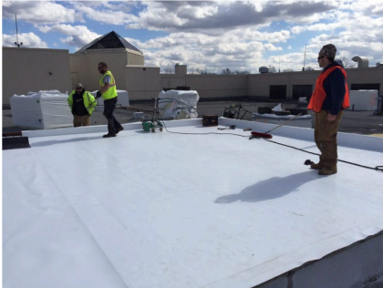
In-progress photo of a TPO roof installation
