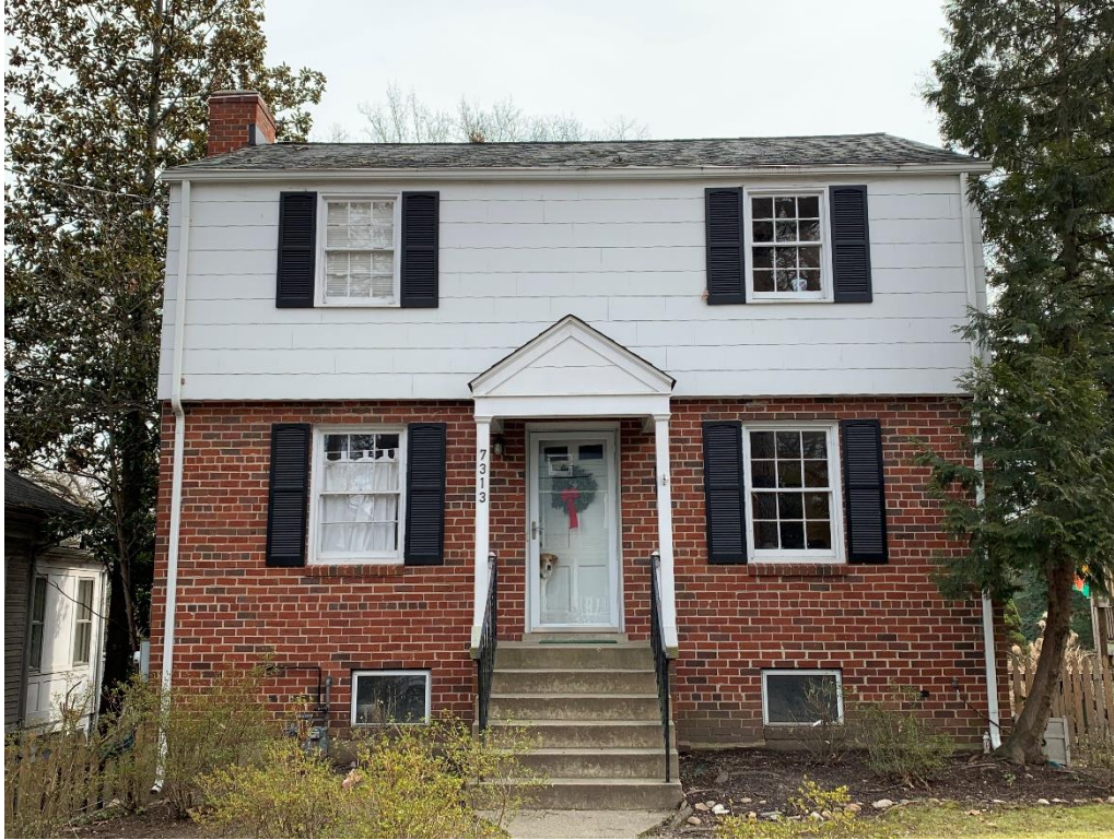
Four of the 9 windows to be replaced.
