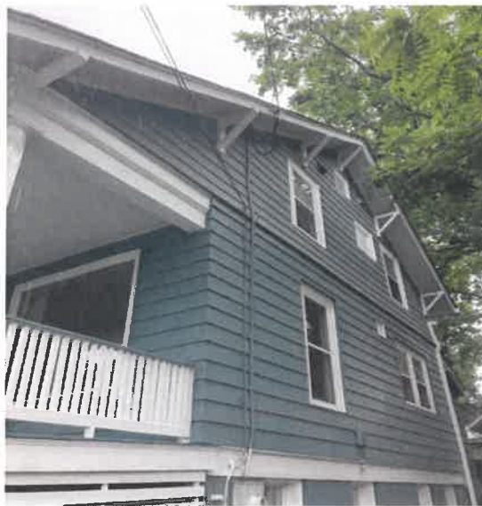
Utility Side Before Installation
