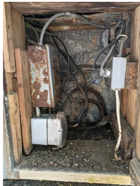
Exterior and interior of electrical equipment cabinet prior to removal of cabinet and deteriorated equipment
