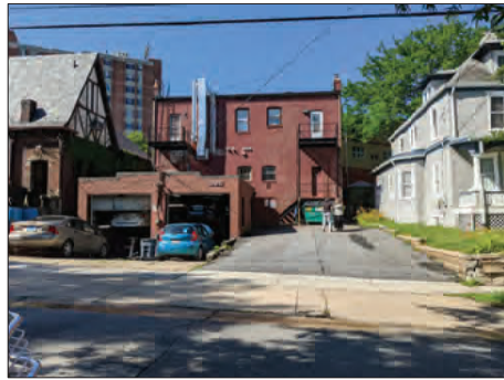
3 EXISTING VIEW FROM TULIP AVENUE A001/ NTS
