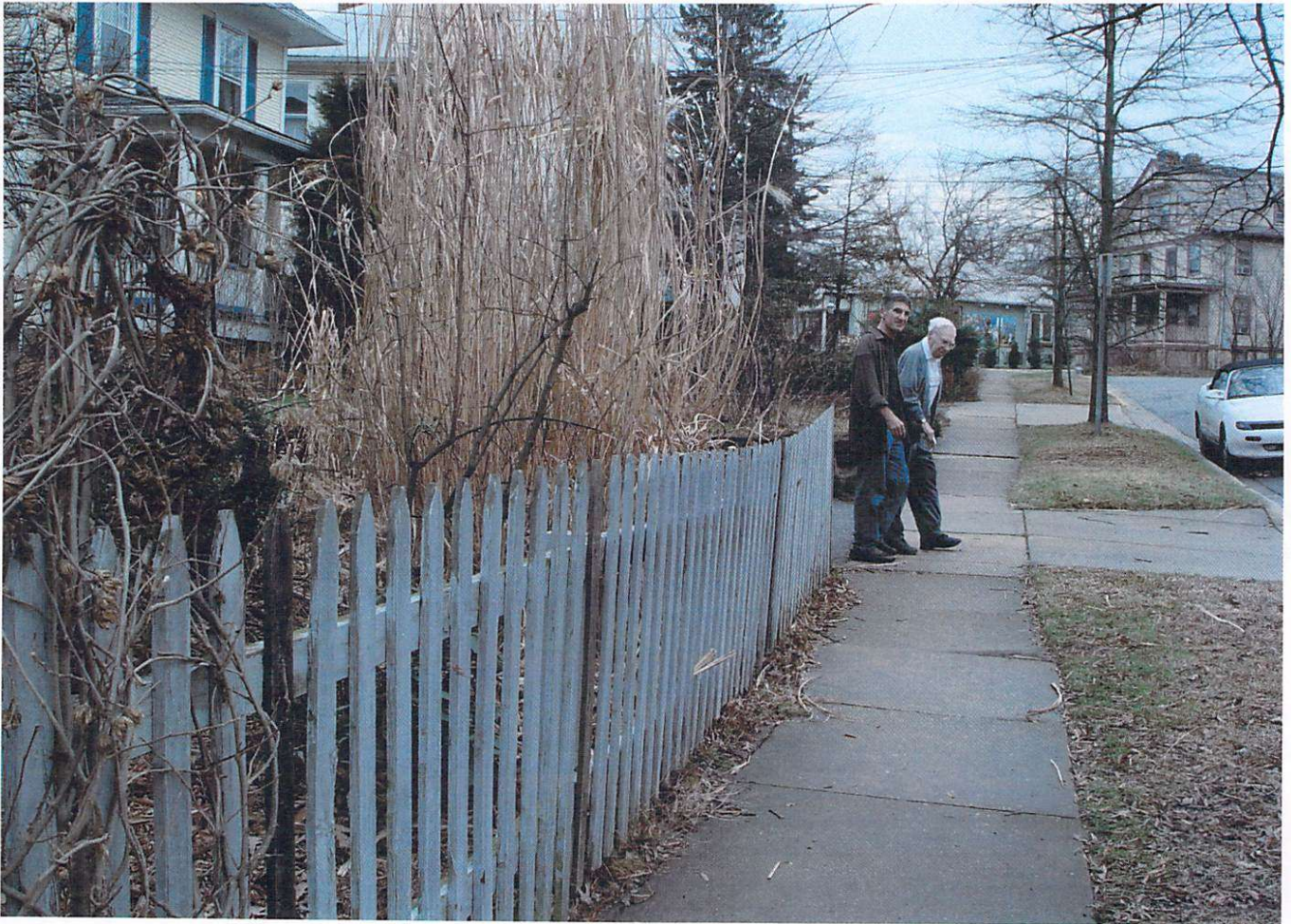
This is the fence to be replaced.
