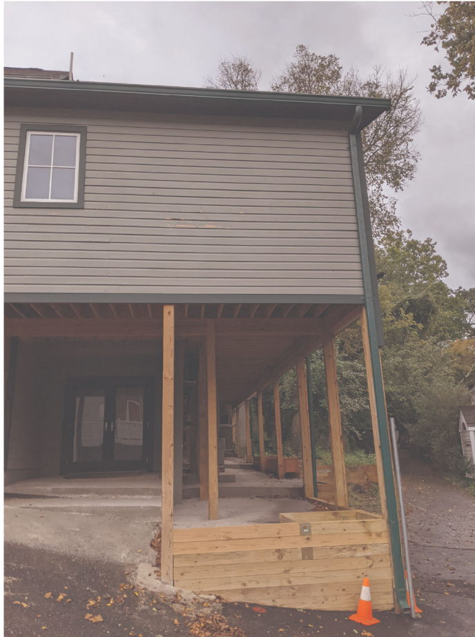
Existing conditions under addition
