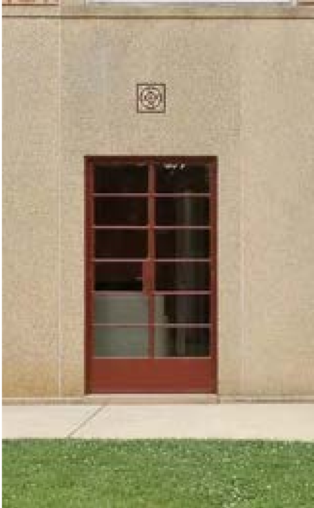
Image of current rear patio door at 9919 Sutherland Road (neighbor):
