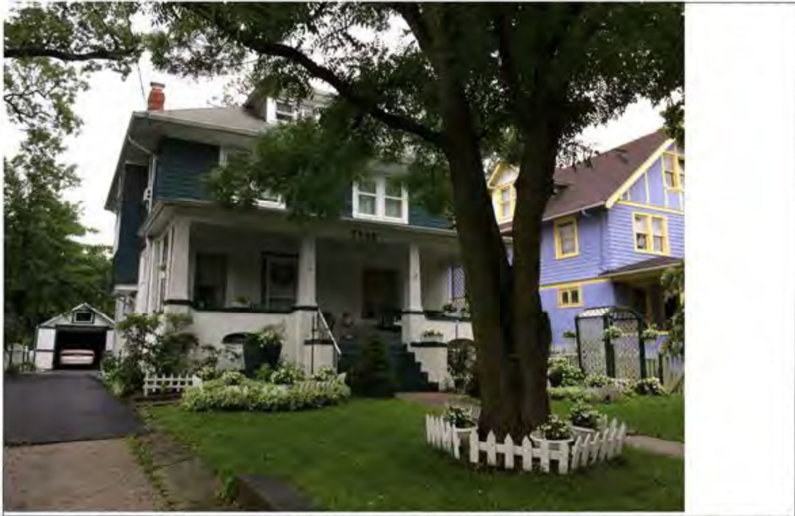
Detail: South adjacent neighbor from public right of way 7115 Carroll
