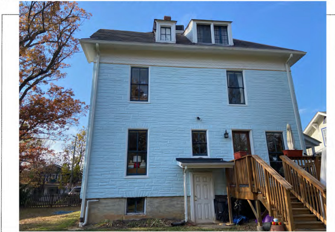
Detail: Rear Facade
