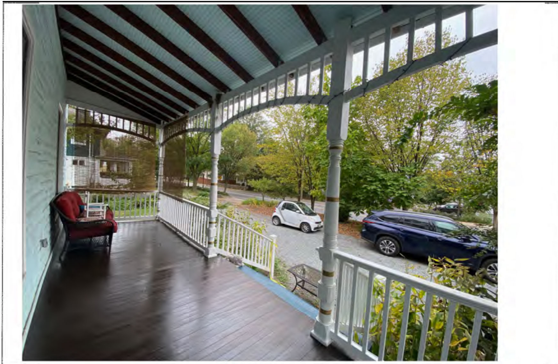
Detail: Front porch (existing)
